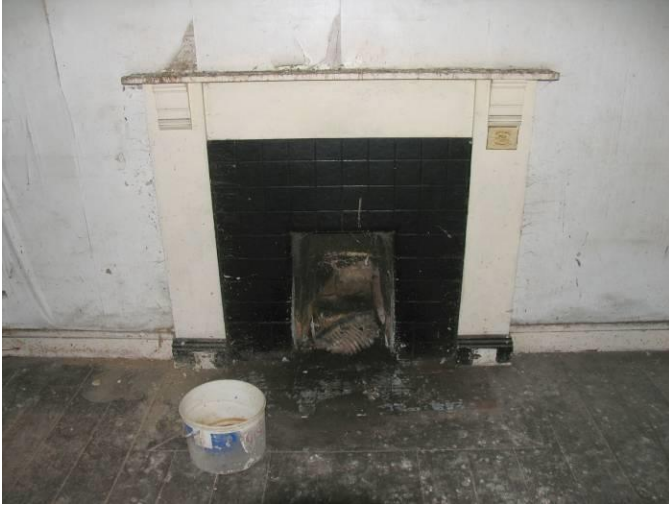
Fireplace to front room
