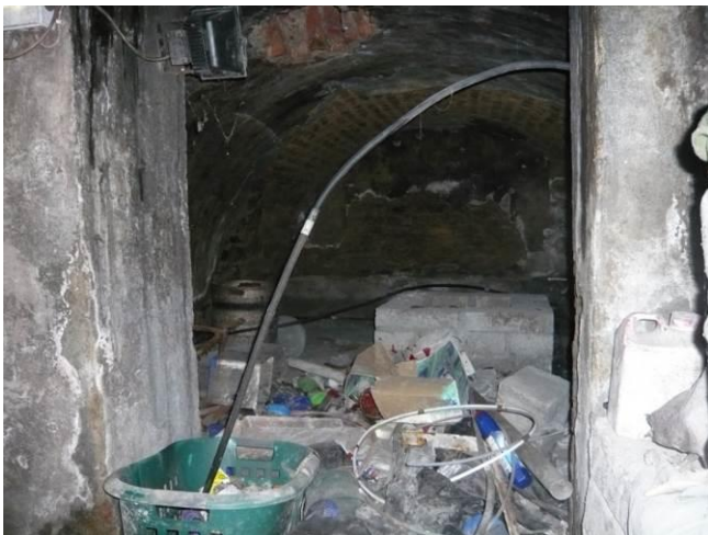
View of one of the two cellars (above) and a typical view of the basement.
