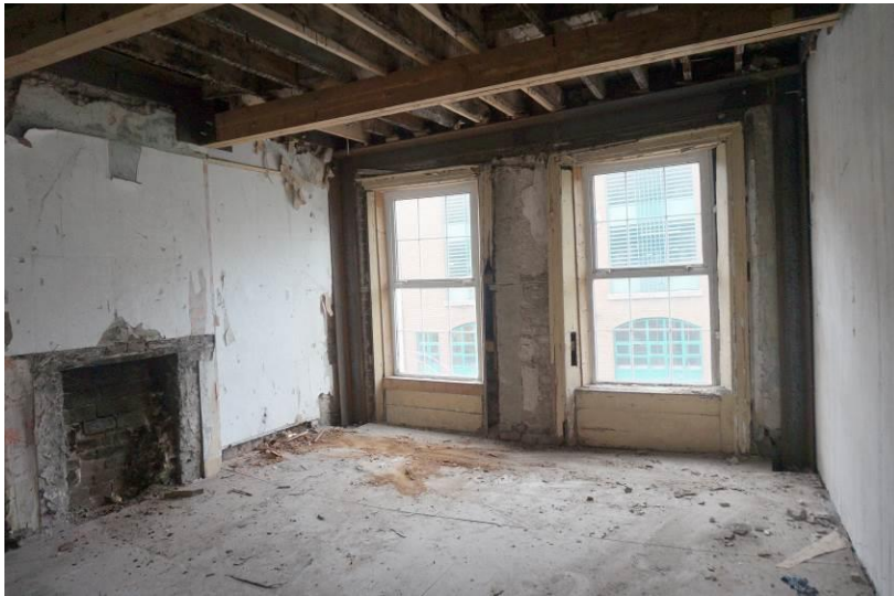
Fig. 2: Front room, second floor, showing stabilisation works.
