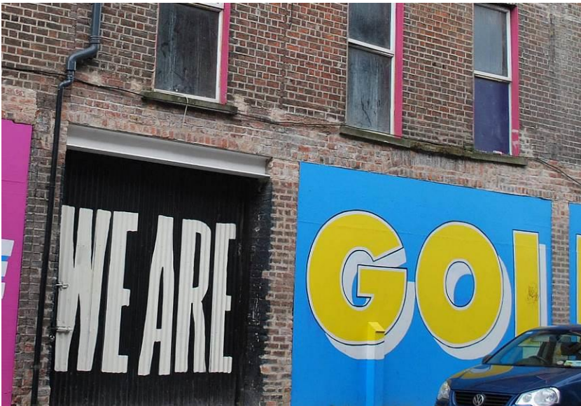
Fig. 4: Beam inserted to carriage archway.
