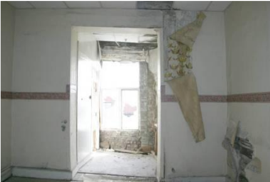
View from rear room through to annex.
