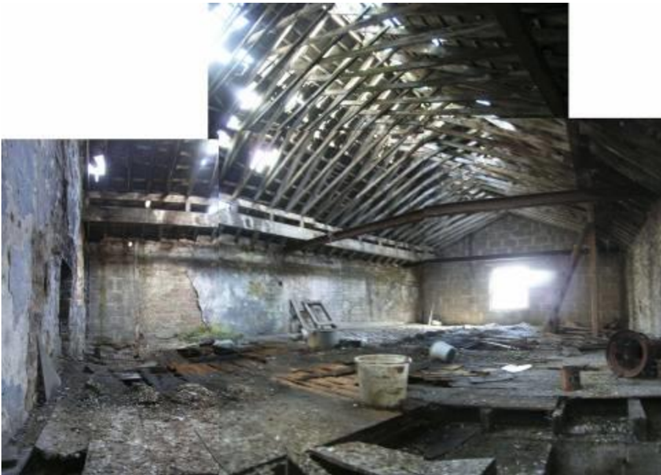
General view of first floor of mews.
