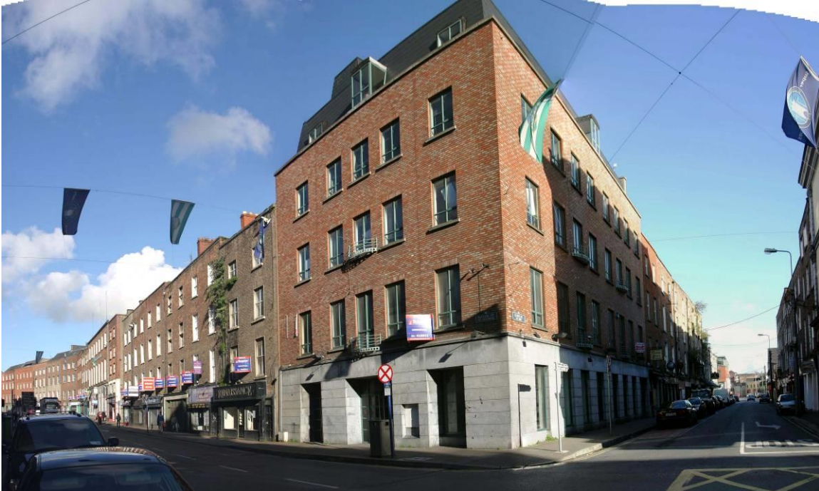
View of 8 Patrick Street, showing both street elevations.
