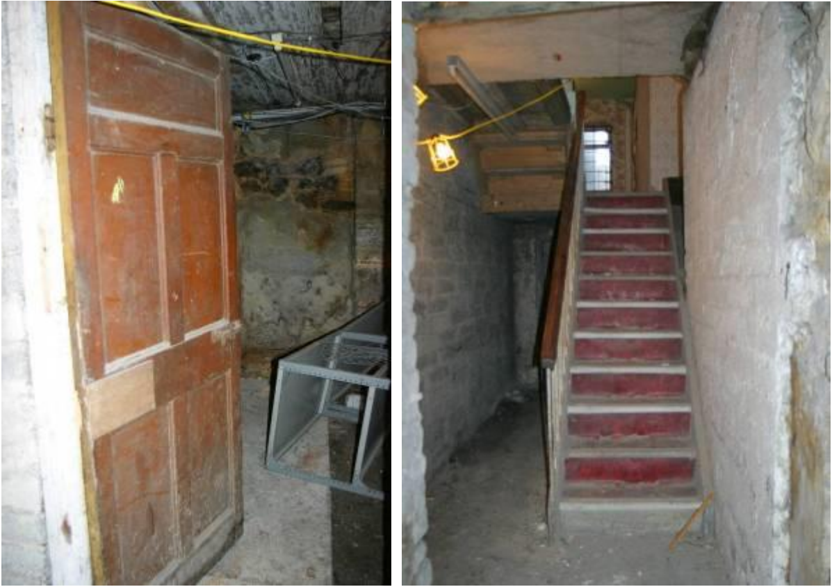
Five panel timber door to rear room of basement (above left) and view of stairs to ground floor (above).
