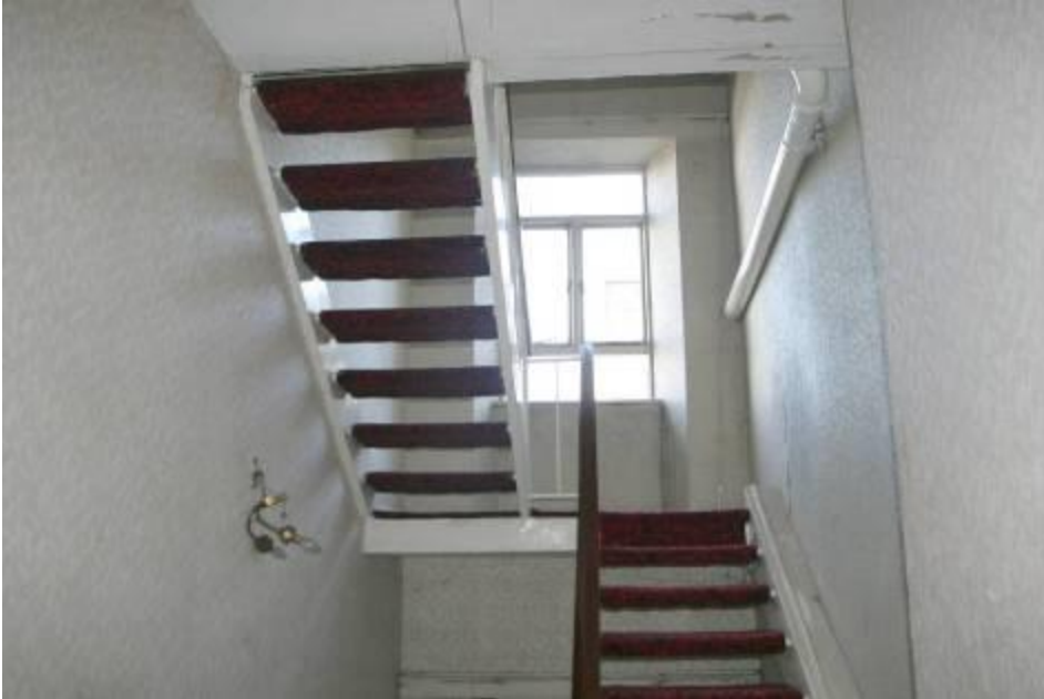
View of replacement staircase.
