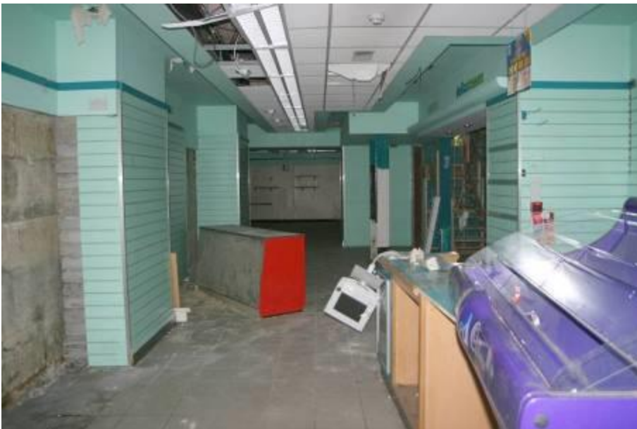
View of the ground floor towards the rear of the building.
