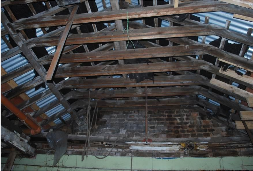
Fig. 5: Corrugated sheets to roof.
