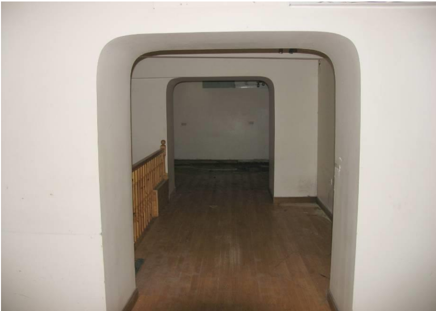
View of the shop area towards the rear of the building.
