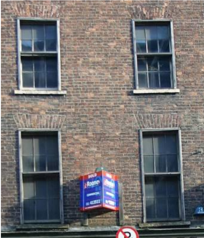
Detail of front elevation showing early timber sash windows (above left) and window to first floor, front room (right).
