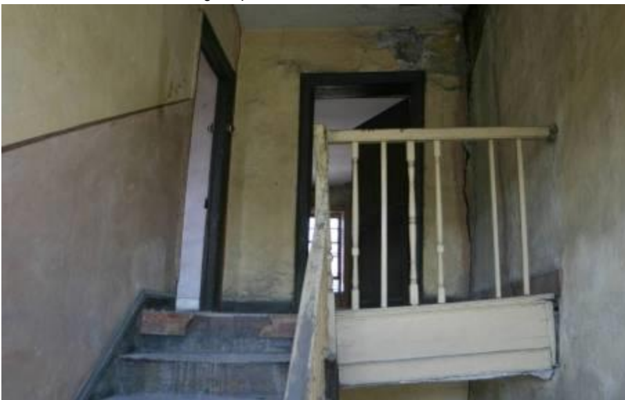
Detail showing top landing and balustrade.
