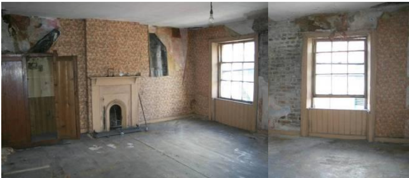
General view of front room, showing windows, fireplace and floor.
