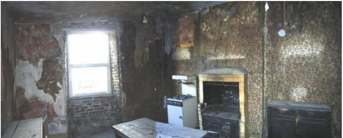
General view of rear room 2
