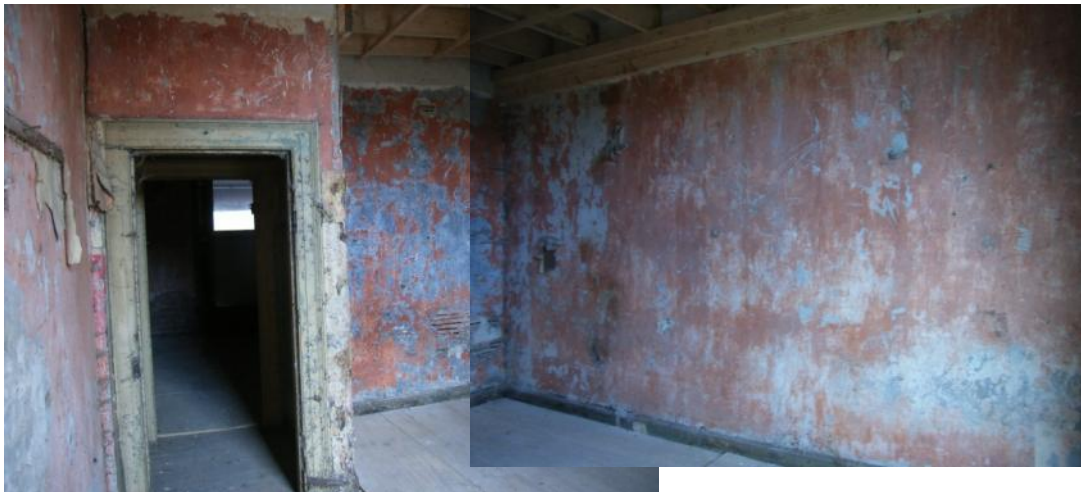
General view of rear room.
