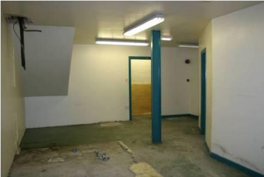
General view of basement.
