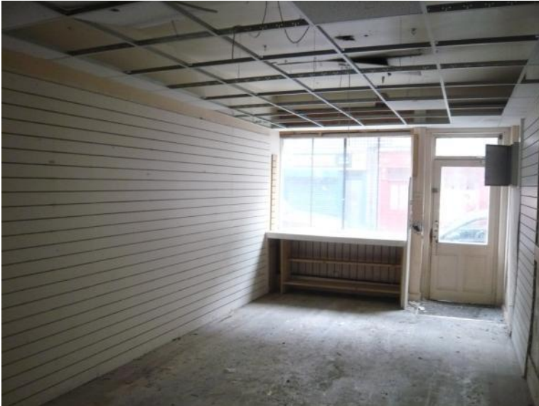
View towards the front of the building.
