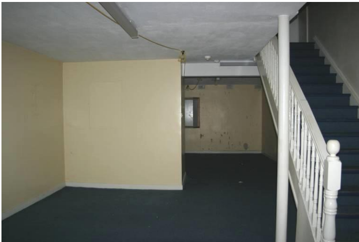
Several views of the basement, showing modern timber staircase.
