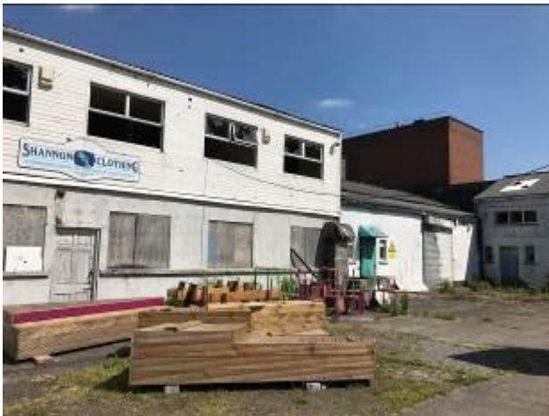
Fig. 1: Northern range of the building.
