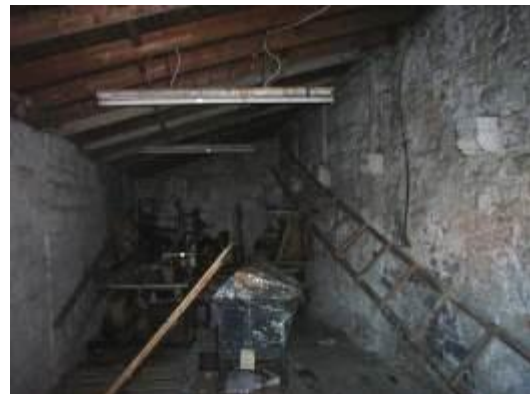
Interior of Lean-to Building
