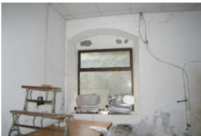
Rear room, showing altered camber headed window opening.
