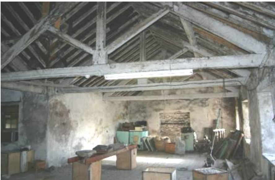
The main area to the second floor, showing roof trusses.
