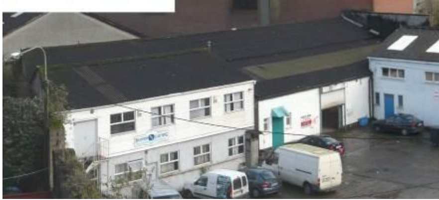
Buildings to Northern Edge of Yard
