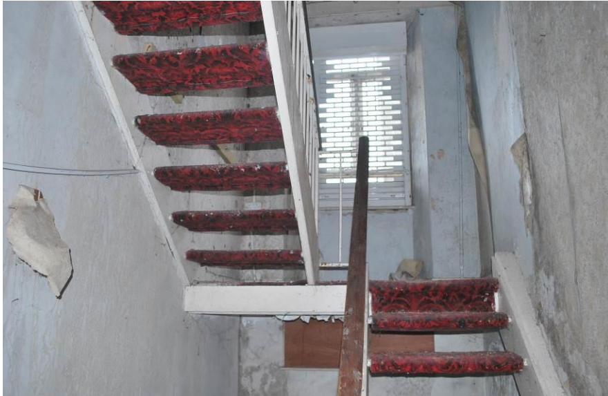
Fig. 3: 20 th century replacement staircase.
