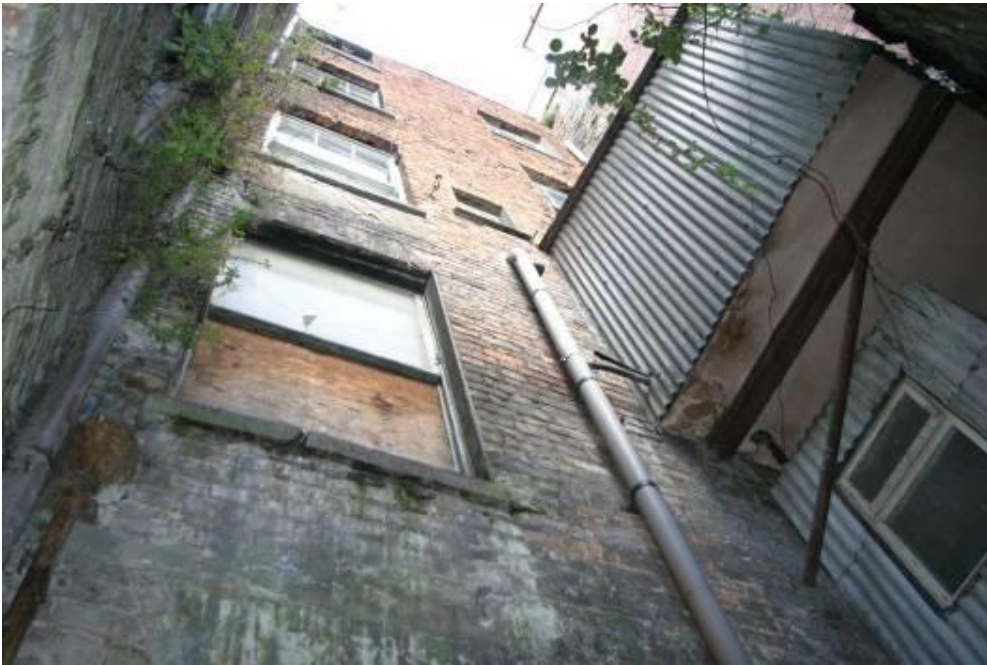
Rear elevation, showing additions leading off half landing of stairs.
