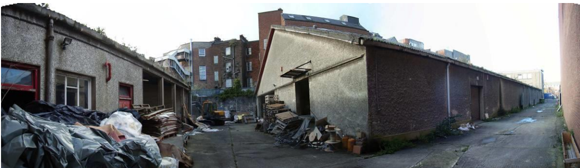
Side and rear of main building to right facing lean-to outbuildings on left of photo.
