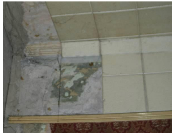
Cornice and picture rail to front room.
