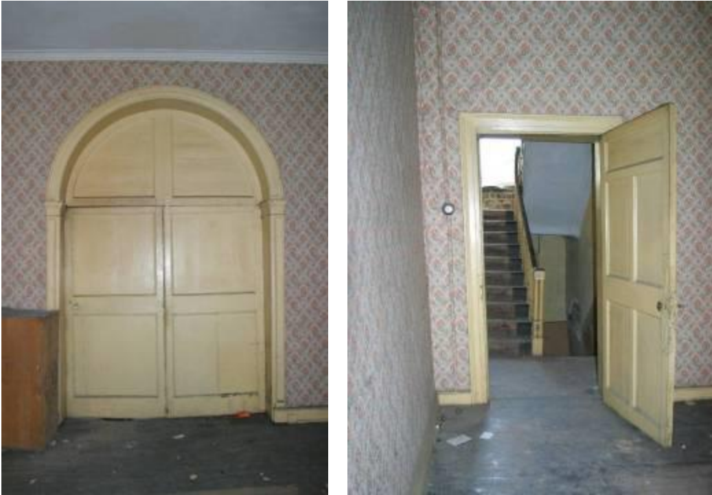
Details from front room, showing double doors connecting to rear room (above left) and panelled door leading to the stairwell (above right).
