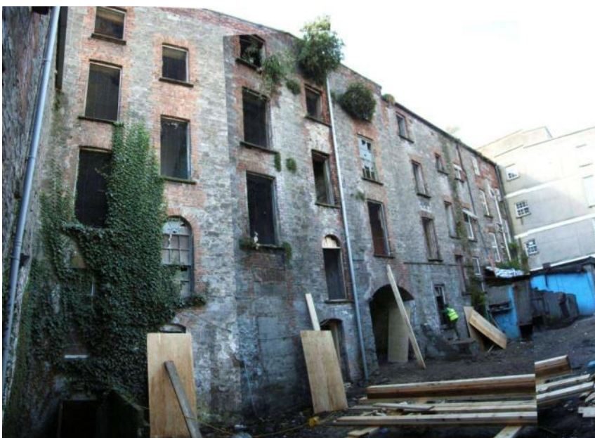
View of the rear of the Ellen Street terrace, showing how few windows remain.
