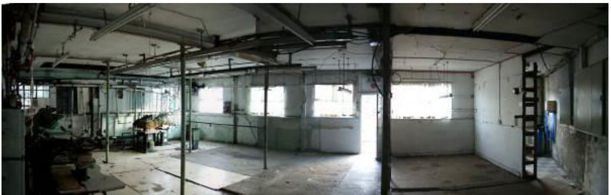
Floor space with intermediate steel columns
