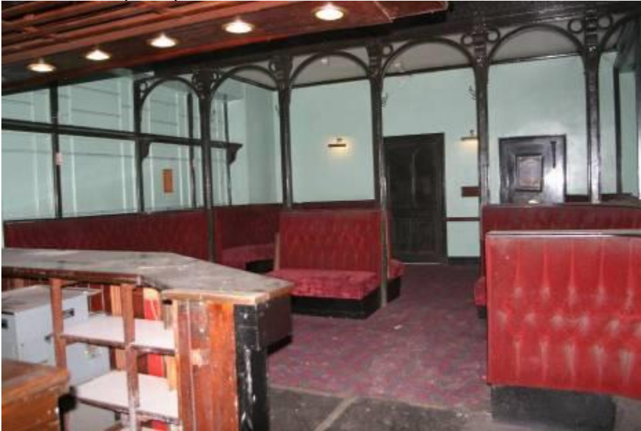
View of area which was likely to have originally been an office, showing timber screen.
