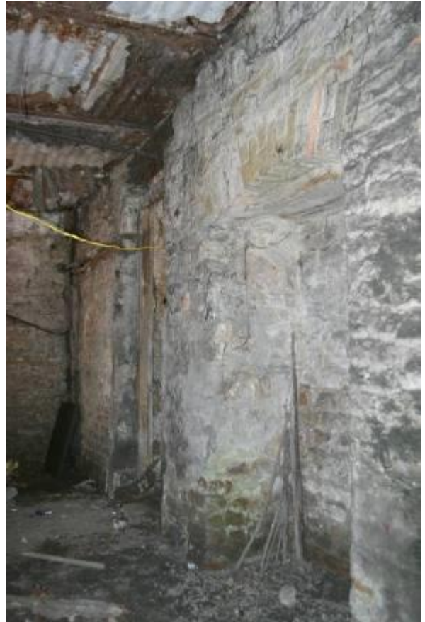
View of area to front of building below the pavement.
