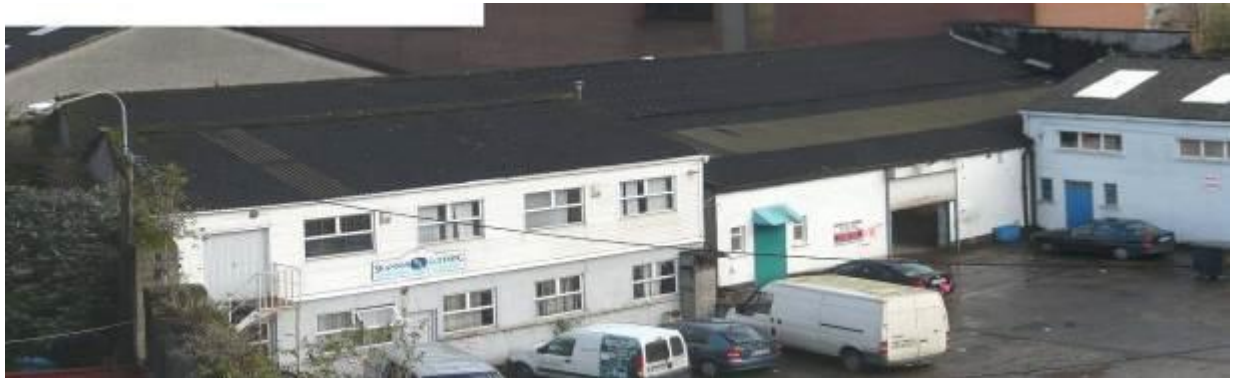
Buildings to Eastern Edge of Yard
