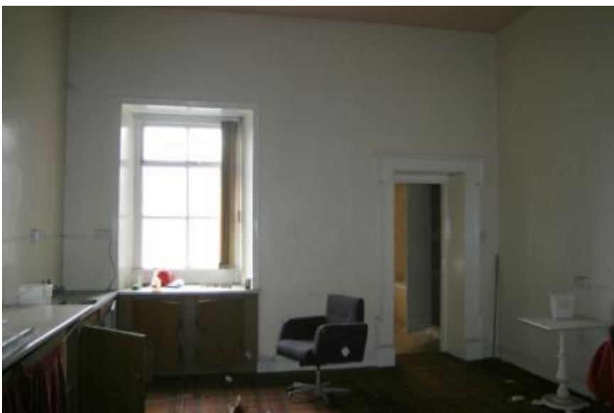
View of rear room showing door through to return.
