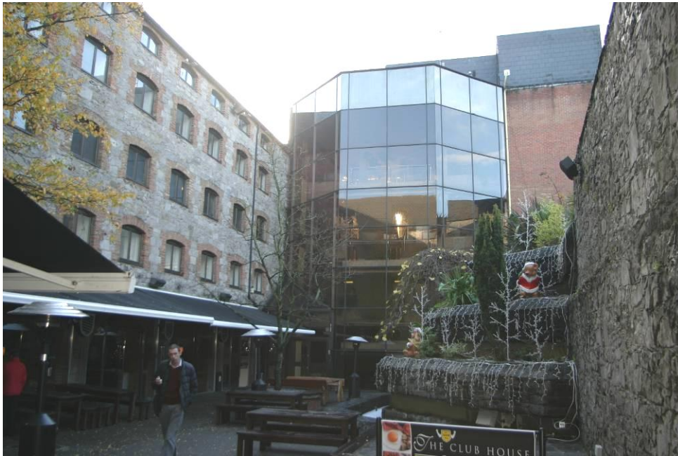
View of south courtyard to granary, showing the 1980s library extension and the remnants of the remainder of the original adjoining warehouse building (right of picture).
