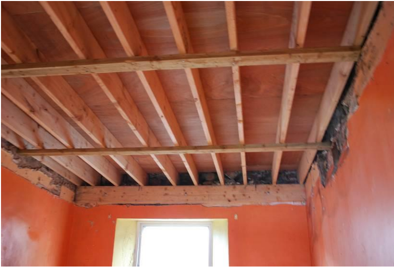
Fig. 3: View of new third floor from second floor, front room.
