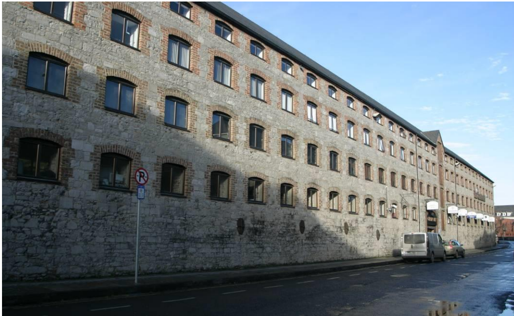
Exterior of the Michael Street elevation, towards Bank Place.
