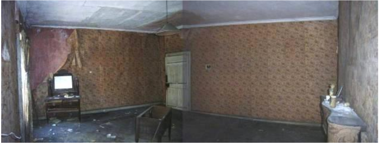
General view of front room 1
