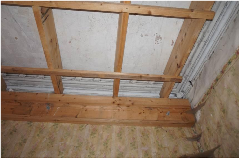
Fig. 3: Floor propped, decorative cornice retained.
