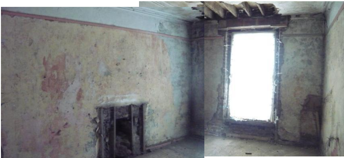
View to front of room showing window.
