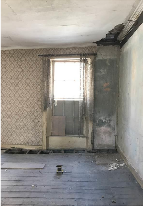
Fig. 3: Front room, first floor.
