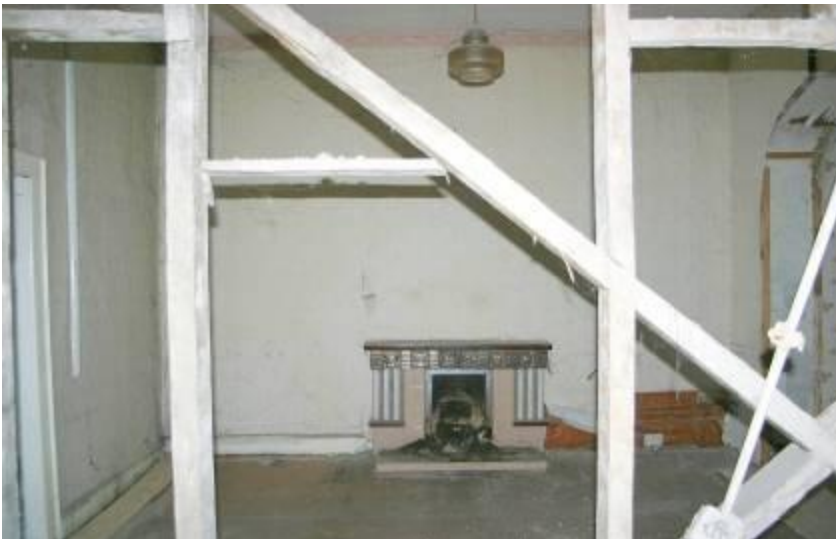
View from hall to rear room, through former brick nogged partition.
