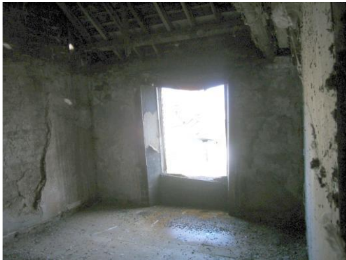
View of rear room.
