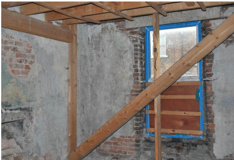
Fig. 1: Temporary structure to prop upper floors, carried out 2007.
