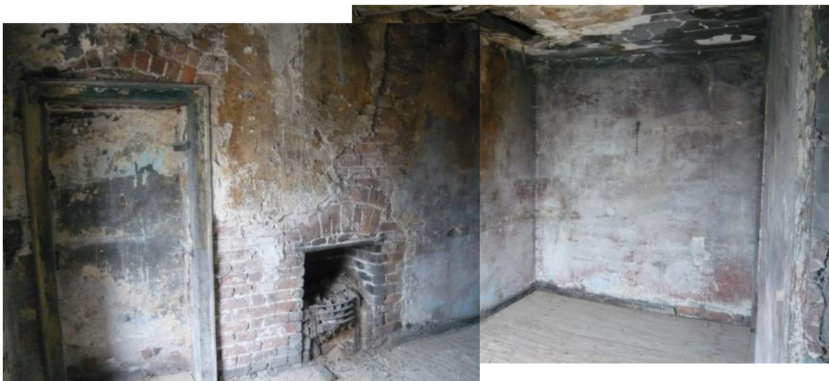
View of rear room, showing fireplace.
