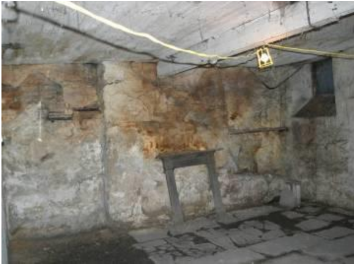
General view of front room, showing flag floor.
