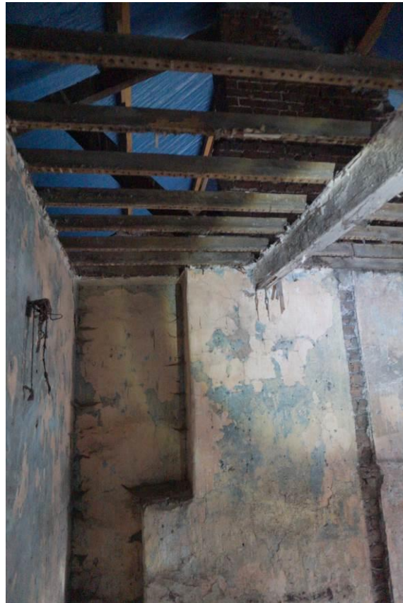
Fig. 5: Second floor, ceiling removed, temporary roof covering.
