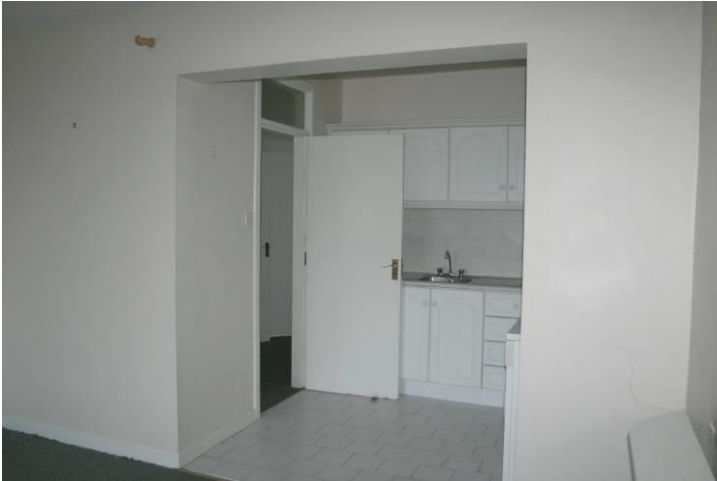
Views of rooms to the third floor, showing the rear room and kitchen (above) and one of the two front bedrooms (above right).
