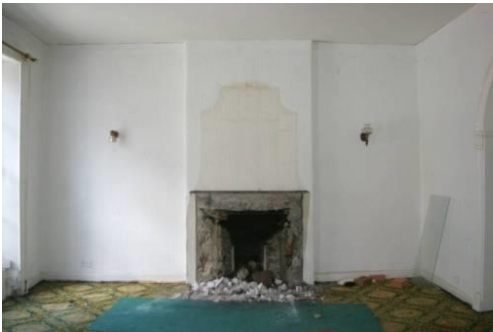
View of front room, showing fireplace with surround removed.
