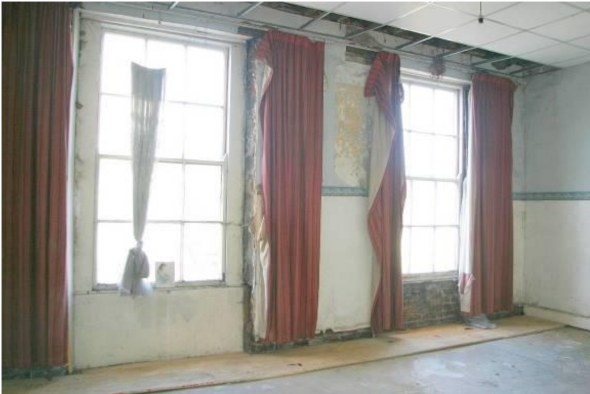
General view of front room, second floor.
