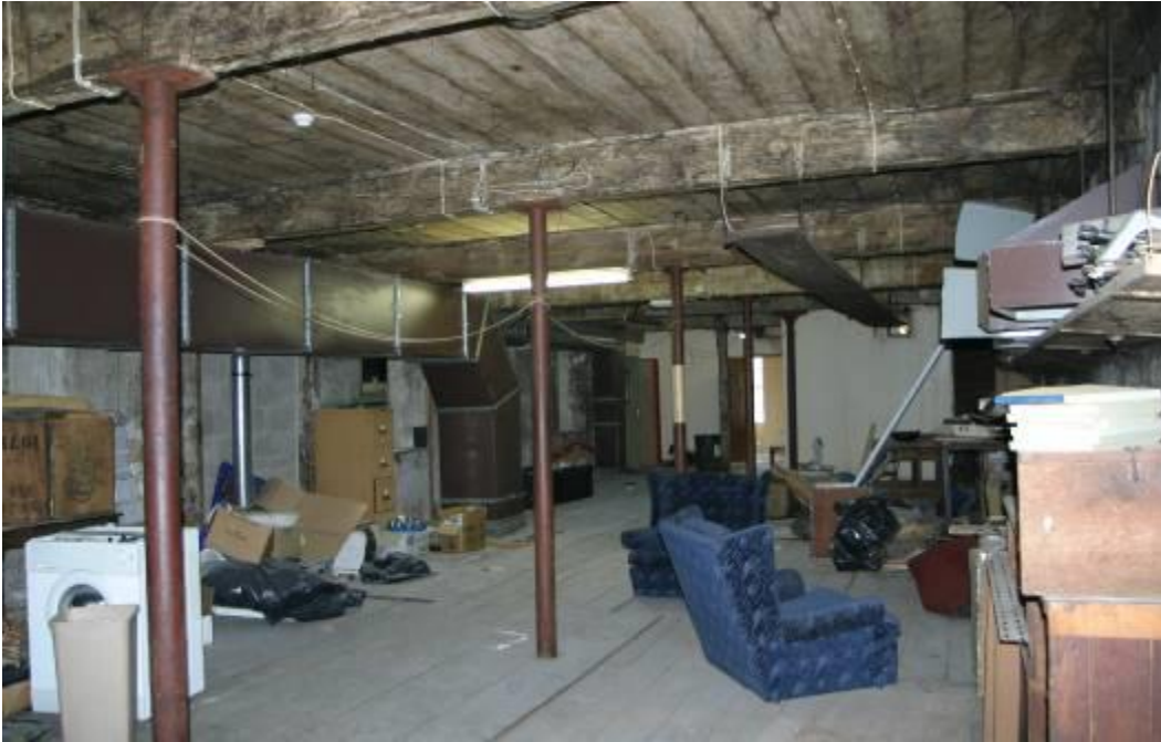
View of the first floor area located above the bar.
