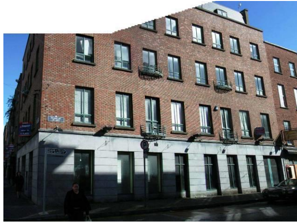
Façade to Ellen Street
