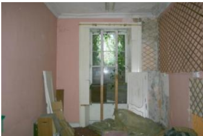
View of rear room, showing ceiling cornice, window and architrave.
