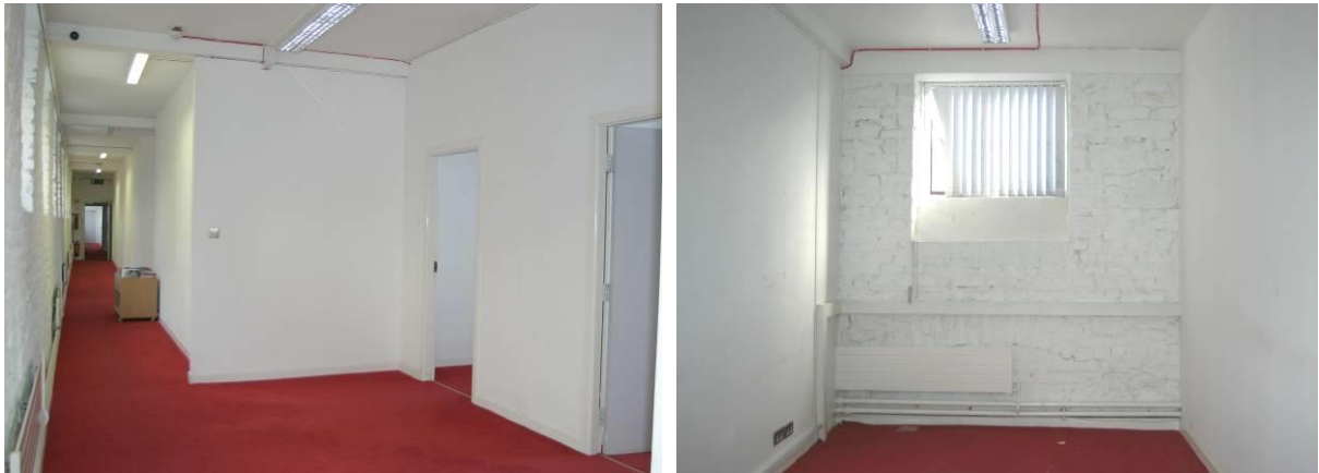
View of corridor and rooms to second floor (above) and a typical office space (above right) showing painted exposed masonry and blocked window opening, showing the change in floors levels of 1980s interventions.
