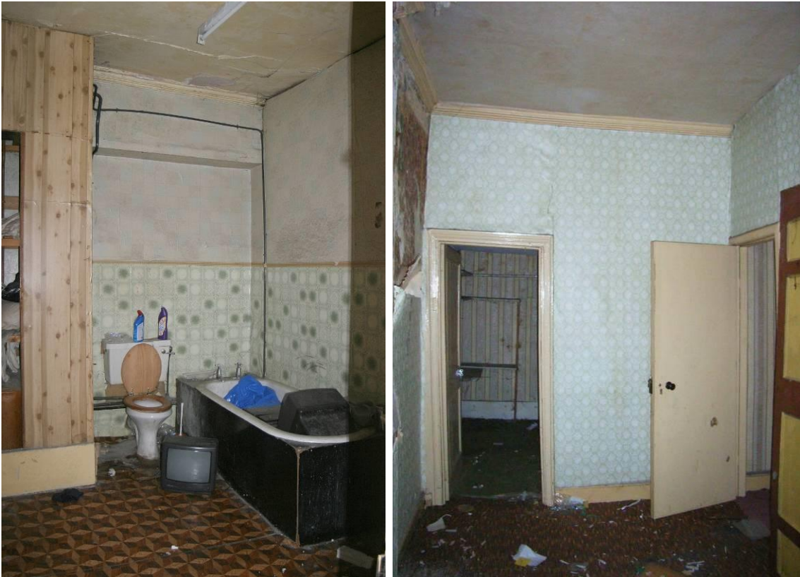
Rear room, second floor, which has been subdivided with a modern stud partition. Note the doorway leading to a small area beneath the stairs (above right).
