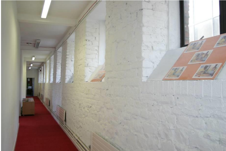
Typical corridor view on second floor.
