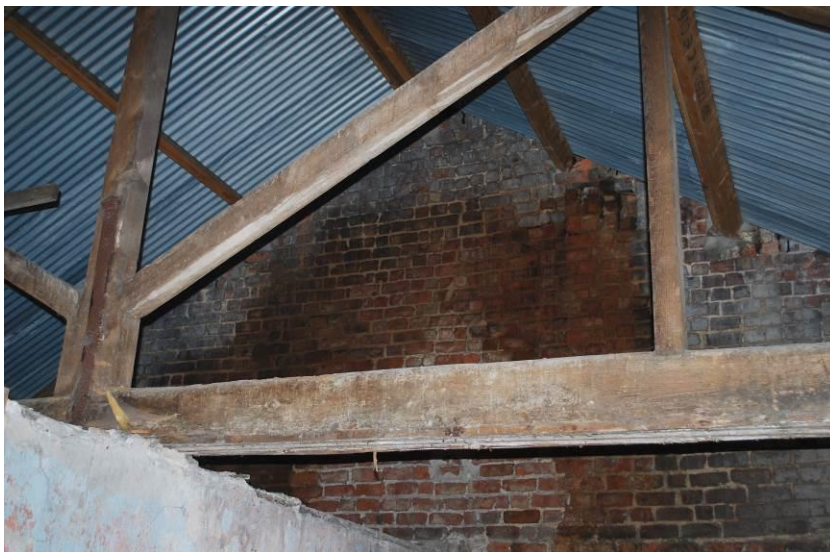
Fig. 2: Ceiling removed and temporary corrugated sheeting to roof.
