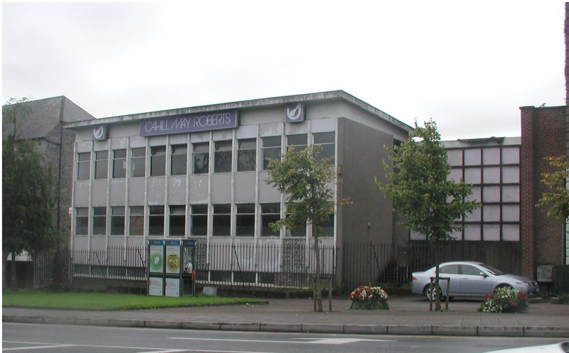
View of front of the building, from Bank Place.
