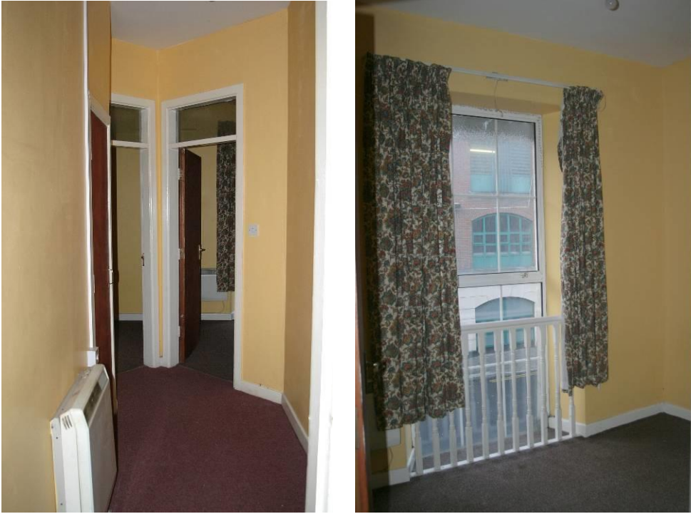
View of front area of first floor, showing the entrances to the two front rooms (above left) and one of the front rooms (above right) showing the altered floor level.
