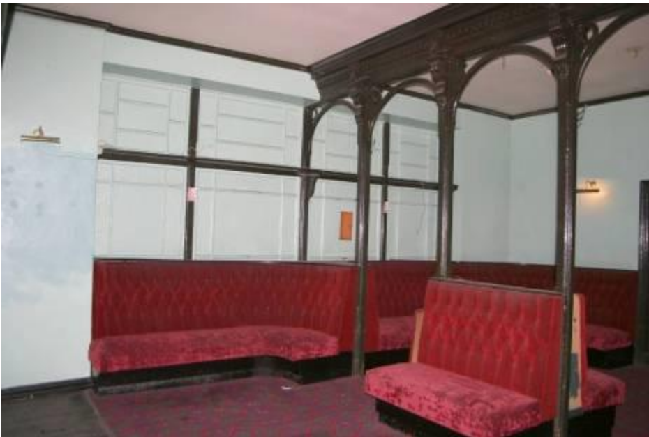
Glazed screen to rear wall of central portion of building, now over painted.
