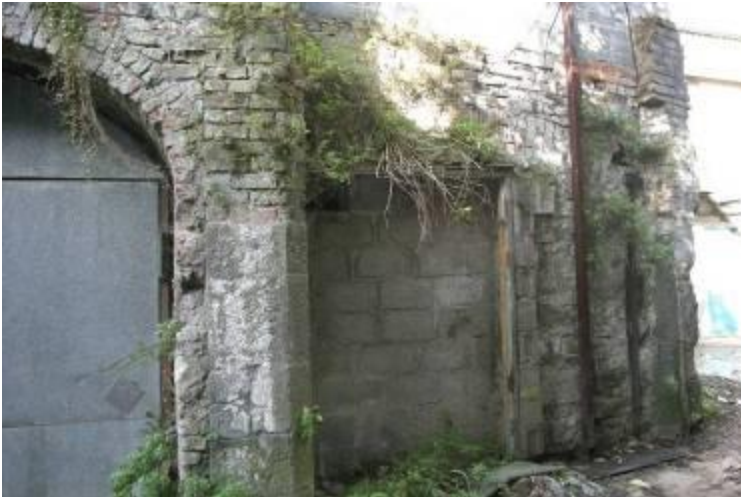
Arched entrance to the outbuilding.
