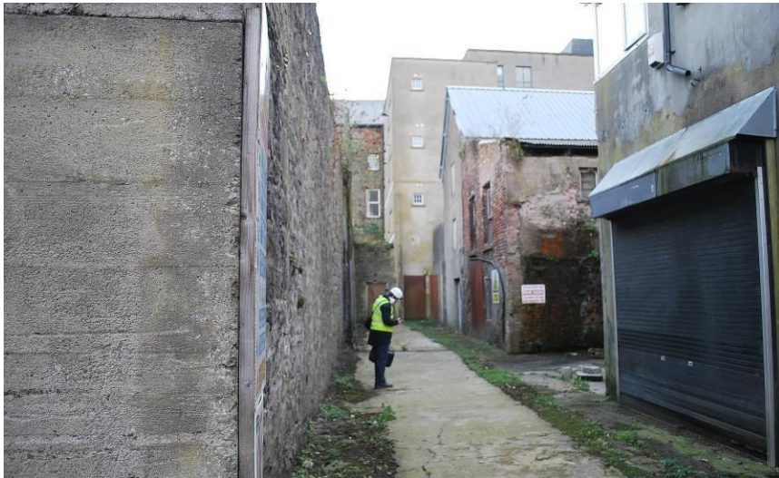
Fig. 1: New corrugated roof to the mews building of 4 Patrick St., as seen from the rear laneway.
