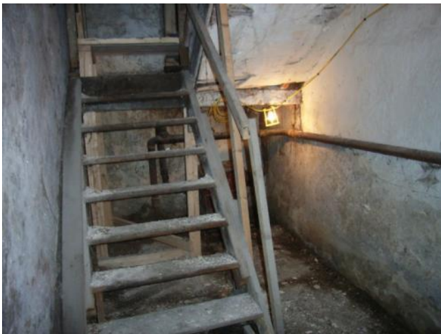
Views of the basement area accessible from No. 7.
