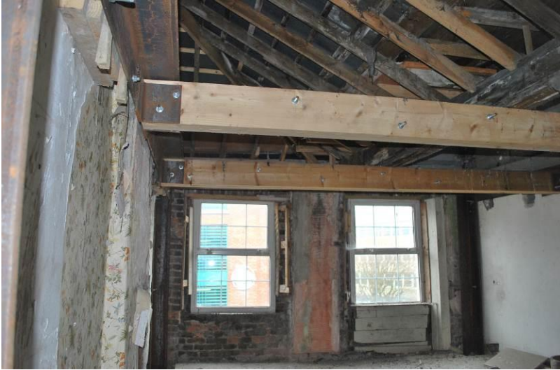
Fig. 5: Second floor, front room, showing central roof beam.
