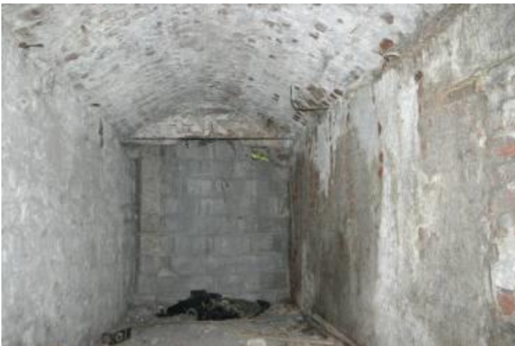
Interior of outbuilding, showing blocked entrance and vaulted ceiling.
