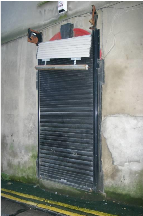
Lugged stone architrave to the original main entrance door on Glover's Lane.
