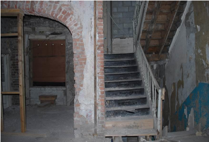
Fig. 6: Staircase, first floor.
