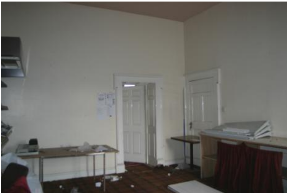
Doors of the rear room, showing the original architraves retained.
