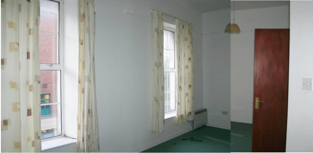
View of the front room, second floor.
