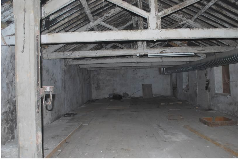
Fig. 3: Exposed roof trusses, top floor.
