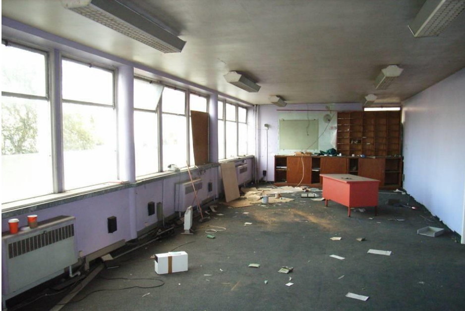
View of typical open plan office area to the front of the building.
