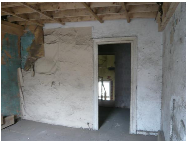
Front room, towards staircase.
