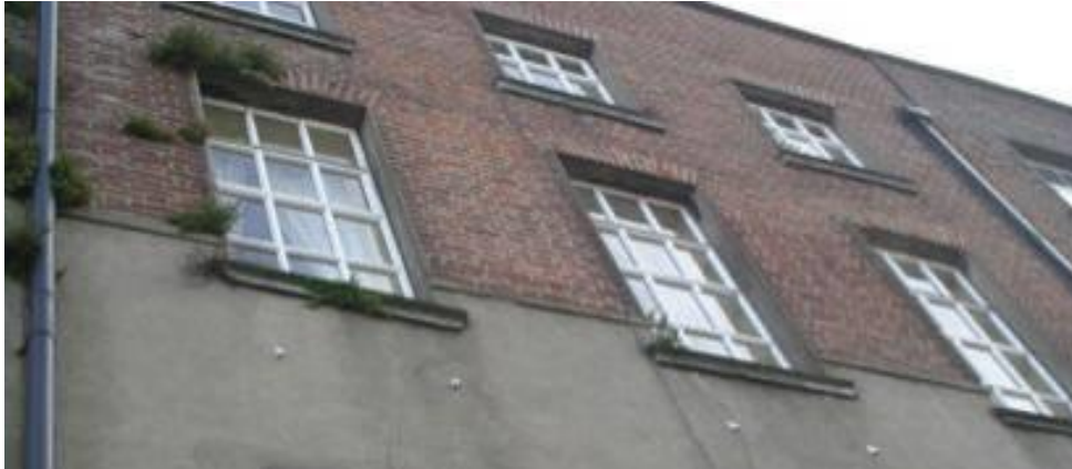
Detail of front elevation showing limestone sills.
