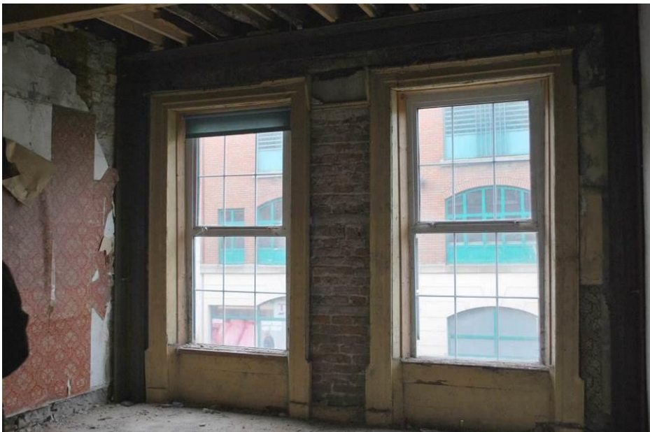
Fig. 1: Front room, first floor, showing lugged architraves to windows.
