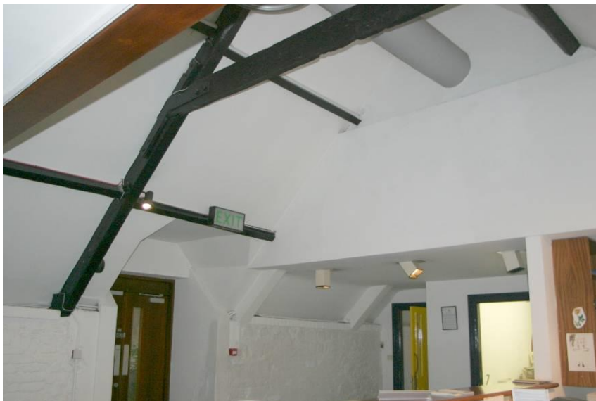
Exposed roof timbers to the reception area.
