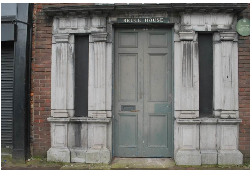
Fig. 2: Limestone door case retained to No. 6 Rutland St.
