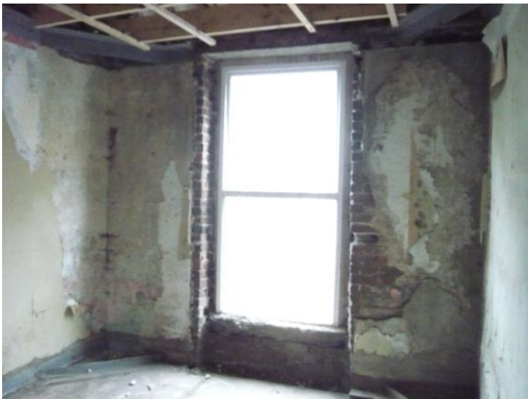
View to front of room showing window.
