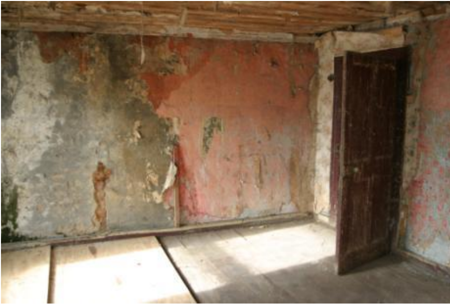
View of front room showing door
