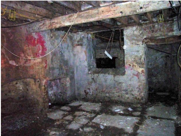
The front room of the basement.
