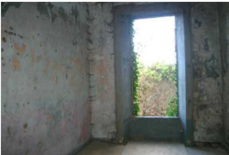
View of rear room, showing window opening.
