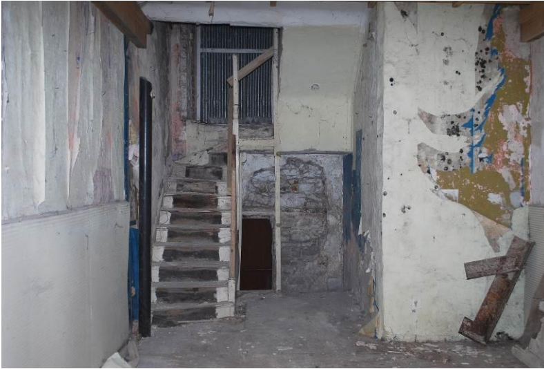
Fig. 3: Staircase (ground to first), and access to basement.
