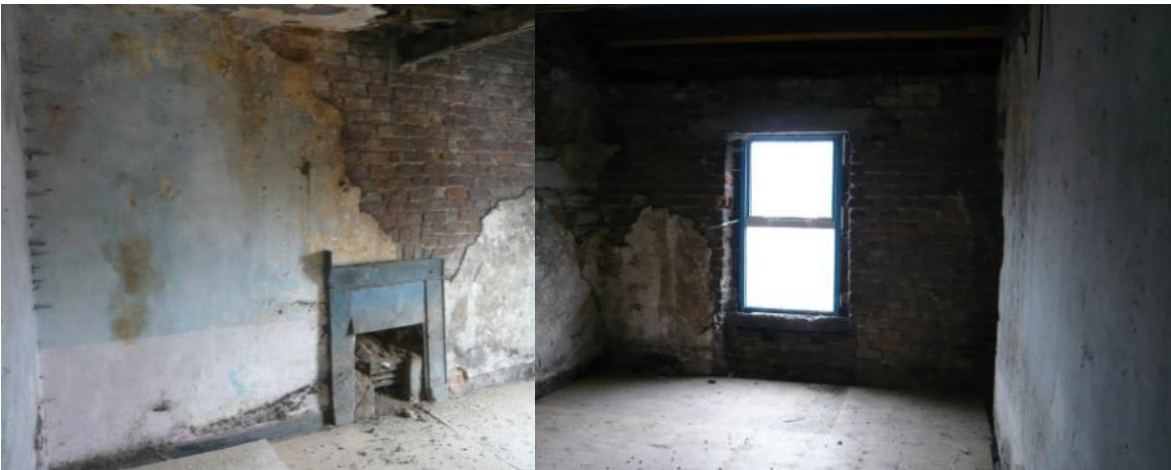
View of front room.
