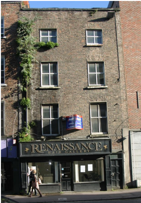
View of front elevation.
