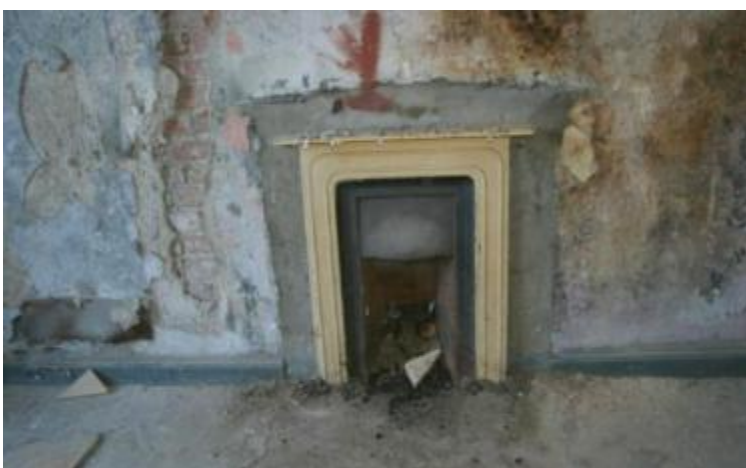
Detail showing fireplace to rear room.
