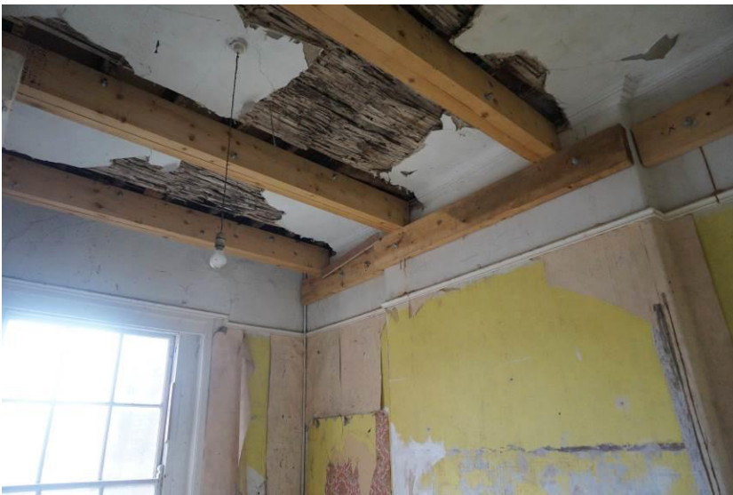
Fig. 4: Second Floor, front room.
