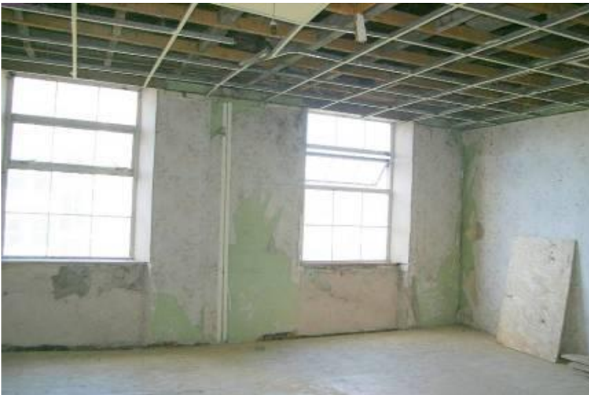
View of front room
