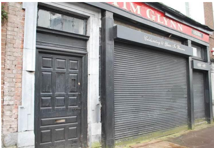
Fig. 1: Shopfront and main entrance door which retains a cut limestone surround.
