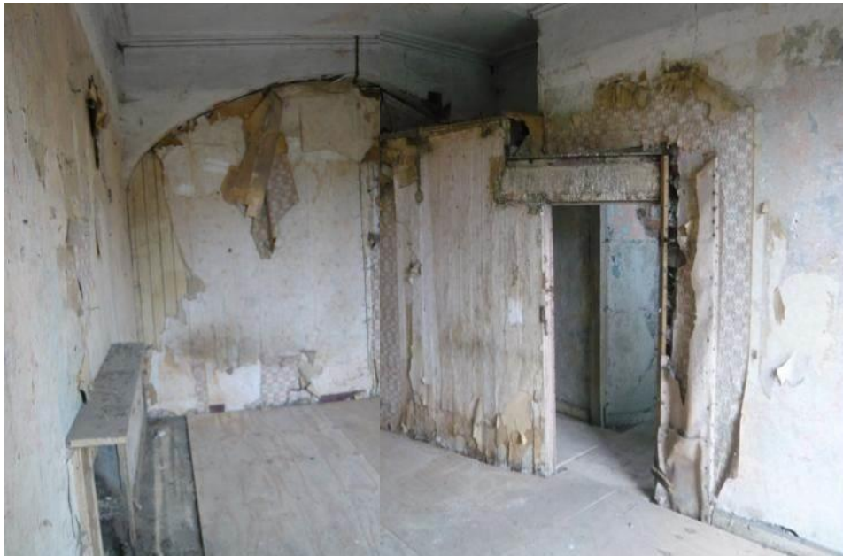
View of the rear room towards the front of the building.
