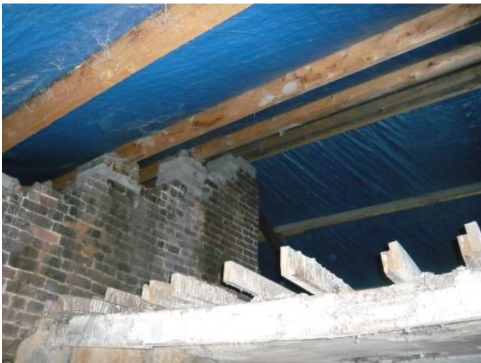
View of roof space where ceiling has been removed.
