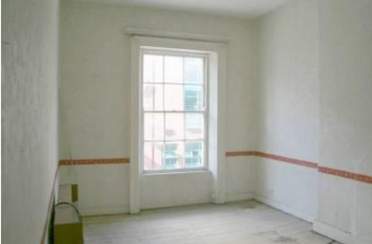
One half of the original front room, showing chimney breast, window architrave and timber floor.
