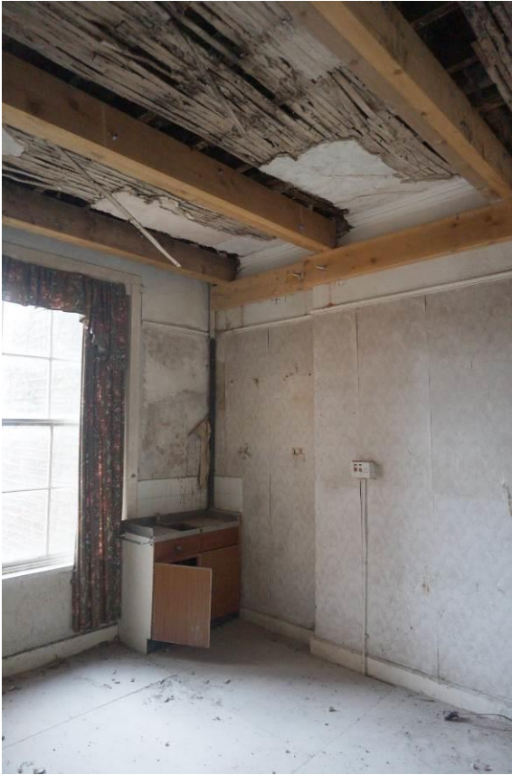
Fig. 6: Rear room, second floor.
