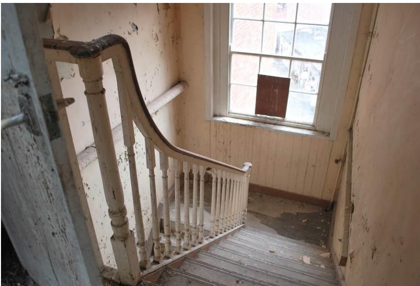
Fig. 8: Staircase, third floor, top landing, showing drop rail balustrade.
