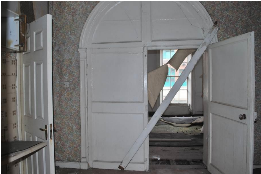
Fig. 4: Original double leaf door in arched opening retained to first floor.
