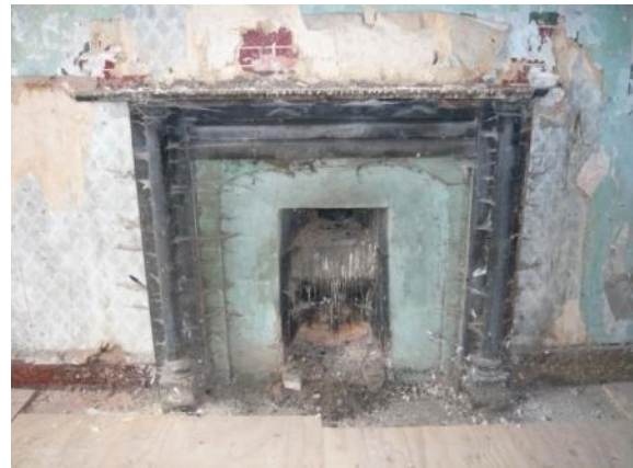
Details showing window architrave and fireplace.
