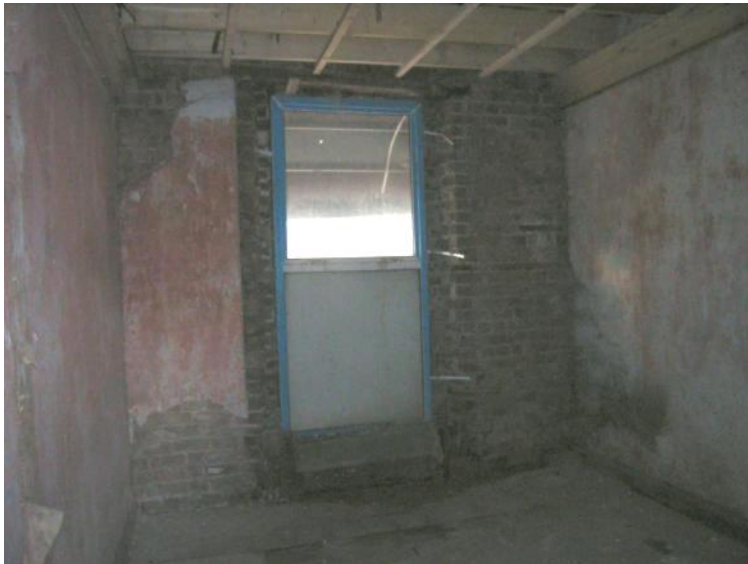
View towards front of building.
