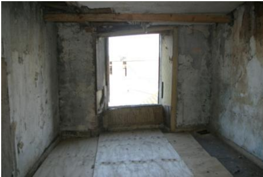
View of rear room
