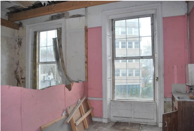
Fig 3. First floor, front room.
