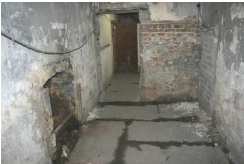
Other area below No. 8 Ellen Street, showing fireplace of original kitchen basement area, now accessed from No.9
