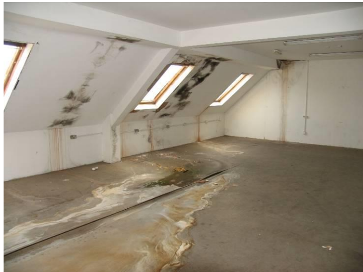
Fourth floor level showing slope in roof line
