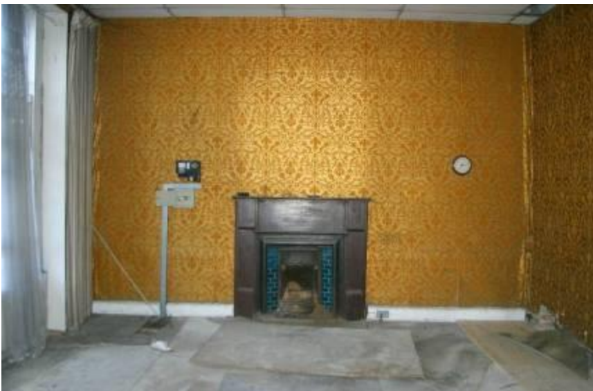
View of front room showing fireplace.
