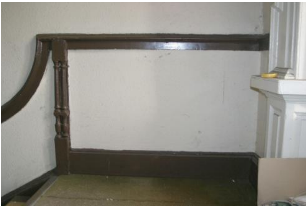
Detail showing the dado rail, complete to the staircase.
