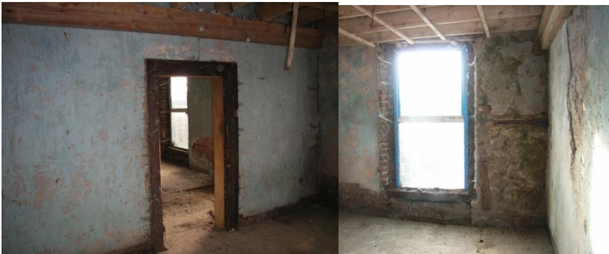
General view of front room.
