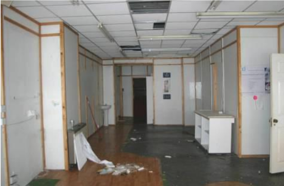
View of shop floor at ground floor level, towards rear of building.
