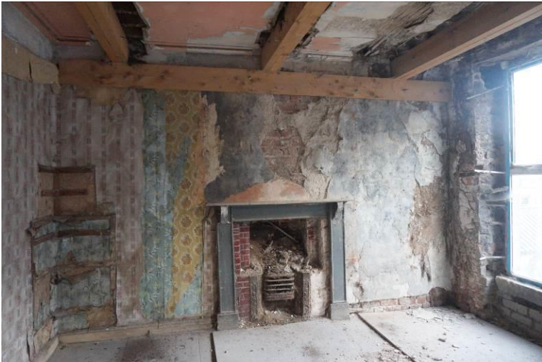
Fig. 5: Second floor, front room.
