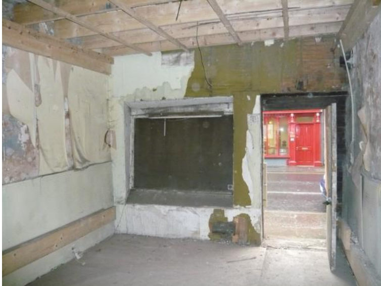
View towards the front of the building.
