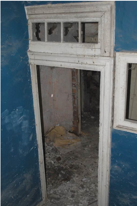
Fig. 4: Partition wall with doorway, off landing, first floor.
