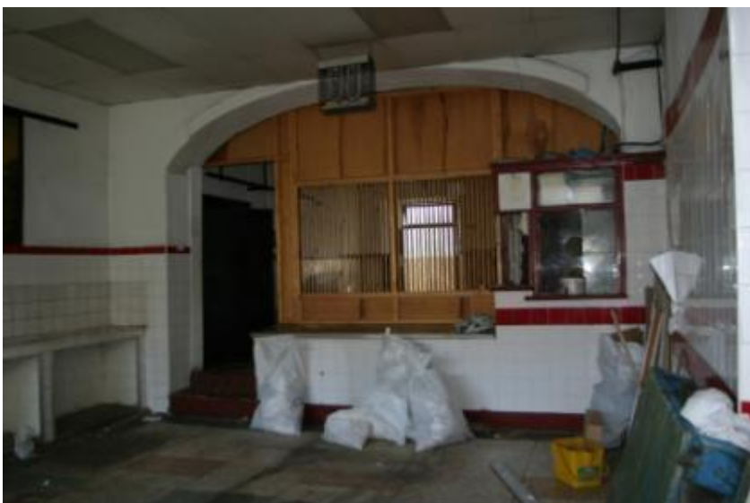
View of arch connecting two rooms of ground floor.
