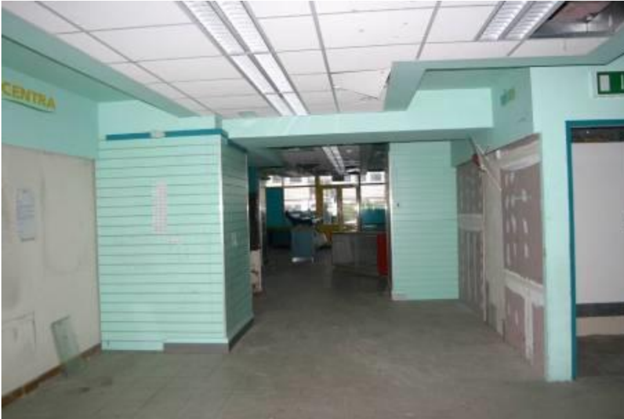
View of ground floor towards the front of the building.
