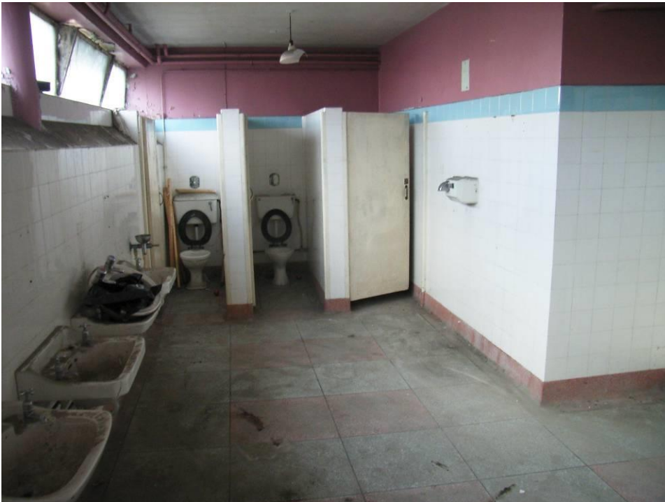
Typical toilet area.
