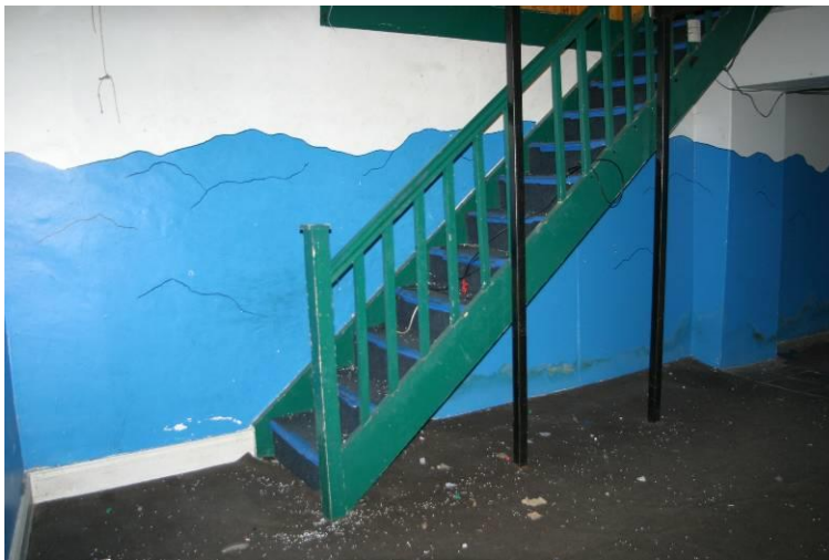
Front room of basement showing access stairs.
