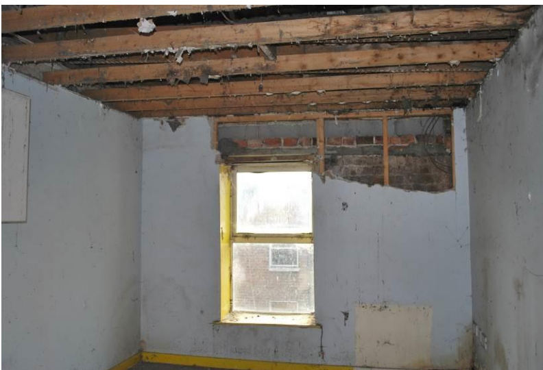
Fig. 4: Front room, third floor, showing repaired parapet.
