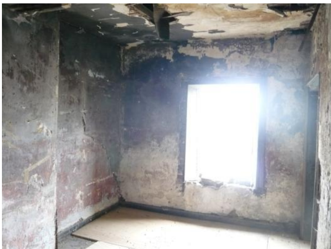
View of rear room showing window.
