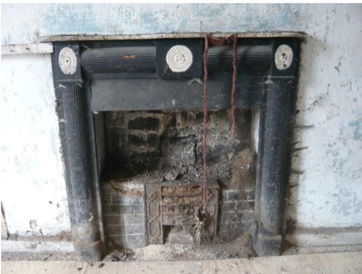
Detail showing fire surround.
