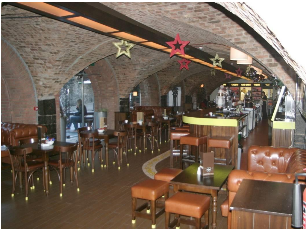
General view of the bar at basement/lower ground floor level, showing the brick vaults (to north).
