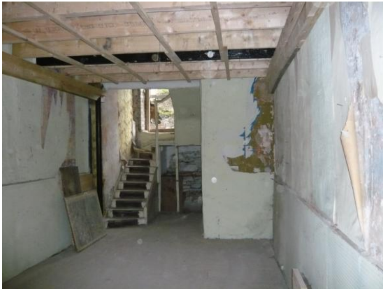
View to the rear, showing staircase.
