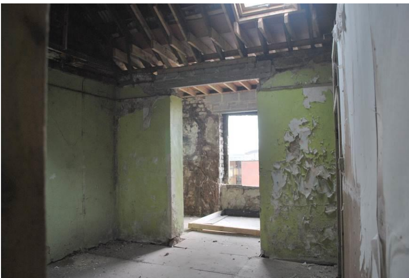
Fig. 4: Rear room, third floor.
