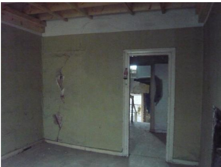
View to rear of room.
