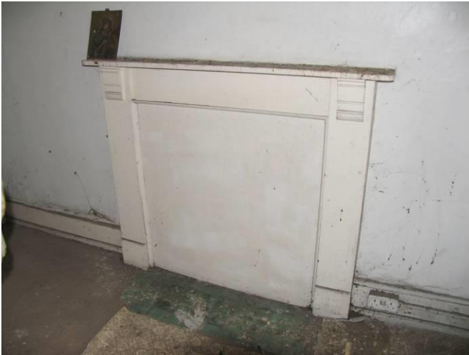
Fireplace to rear room
