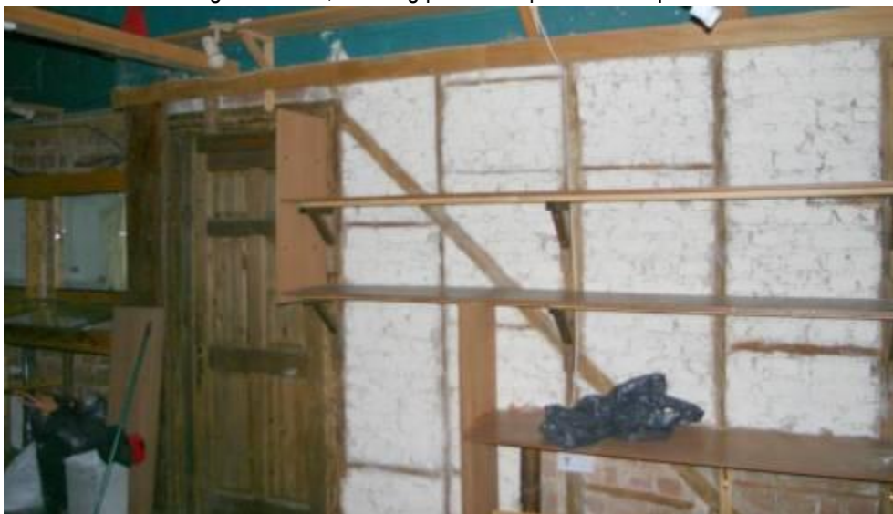
Brick nogged wall between rear room of retail area and stairwell.
