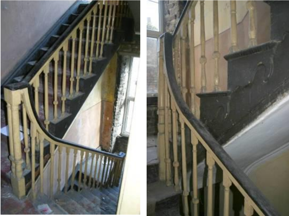
Details of staircase, showing drop handrail, carved tread ends and cornice to soffit.
