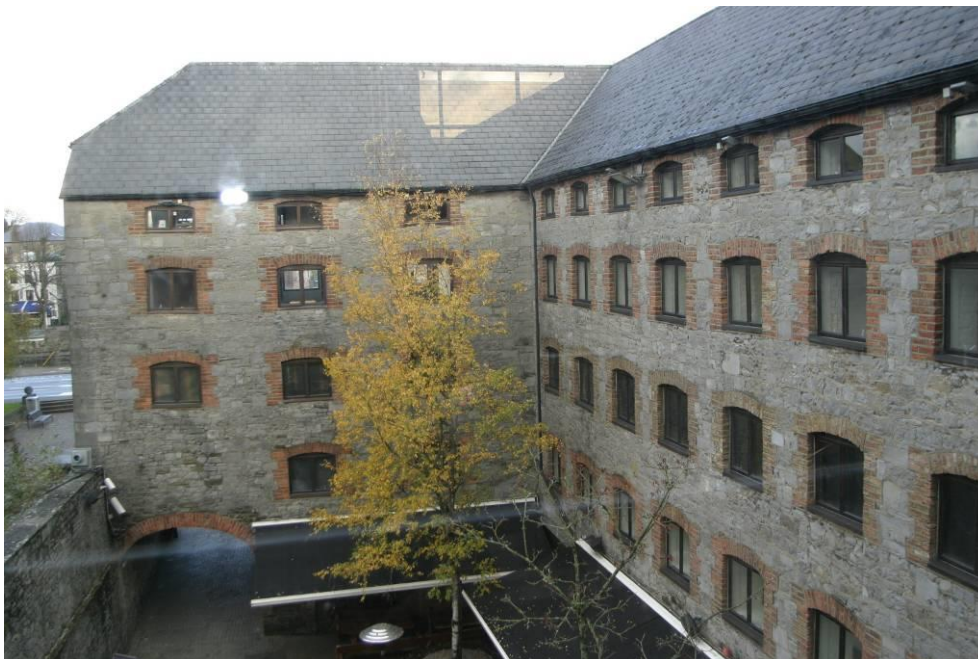
View from stairwell of library, to the west, showing the south and east facing elevations of the granary.
