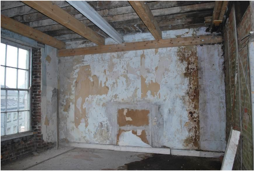
Fig. 2: Second floor, front room.
