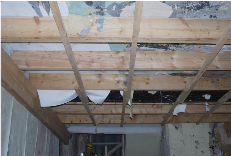
Fig. 1: Works to reinforce floors (ceiling to ground floor).
