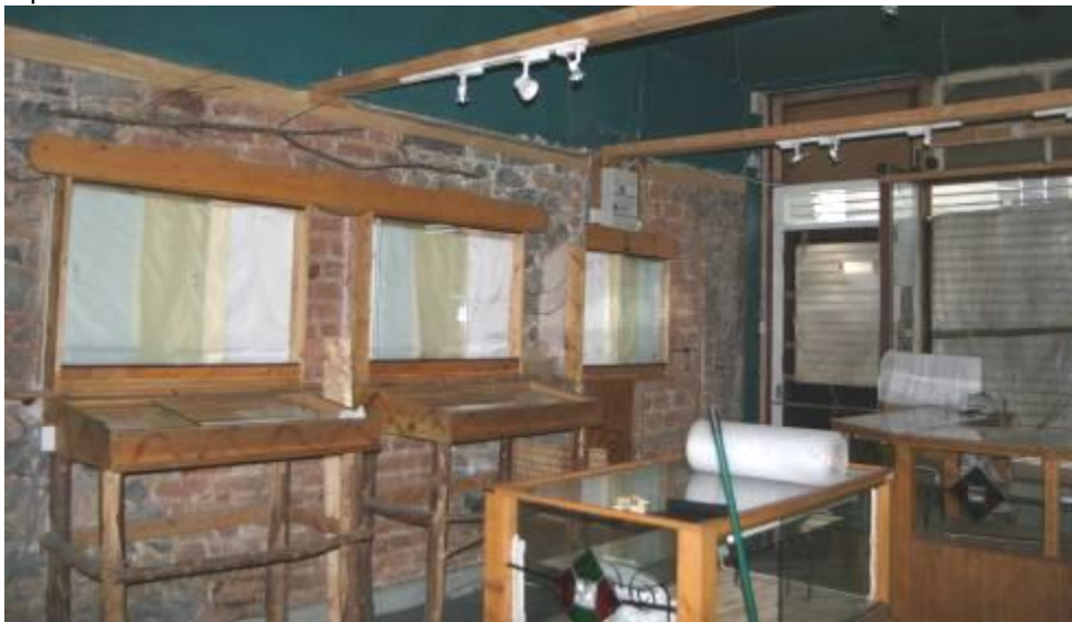
View of retail area to ground floor, showing part of shopfront and exposed walls.
