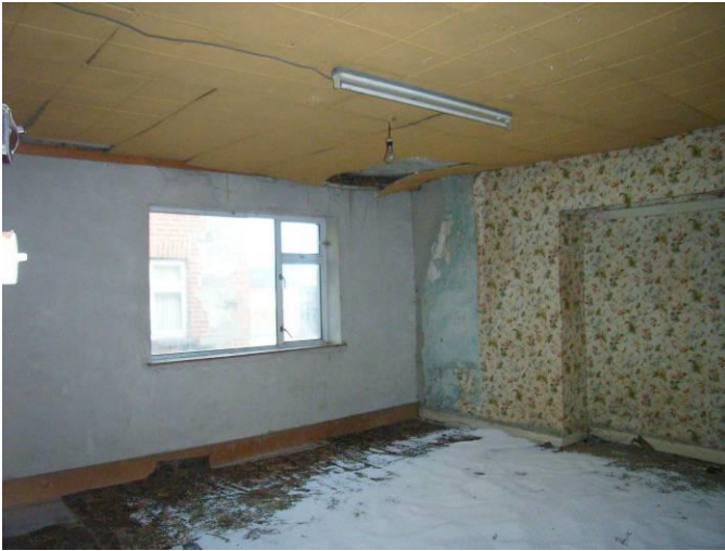
Views of rear room, showing blocked opening to rear wall and panelled door.
