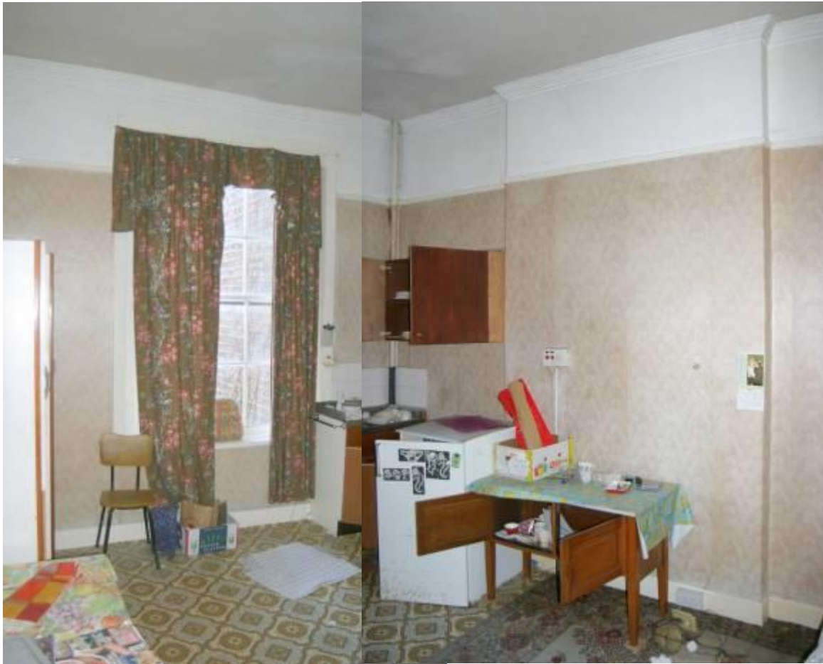
View of rear room, showing chimney breast, cornice and picture rail.
