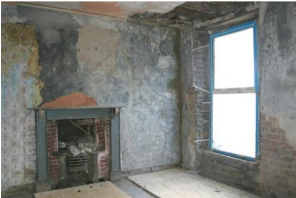
General view of front room showing fireplace with raised hearth.
