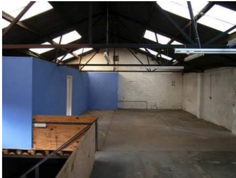
View above mezzanine showing roof
