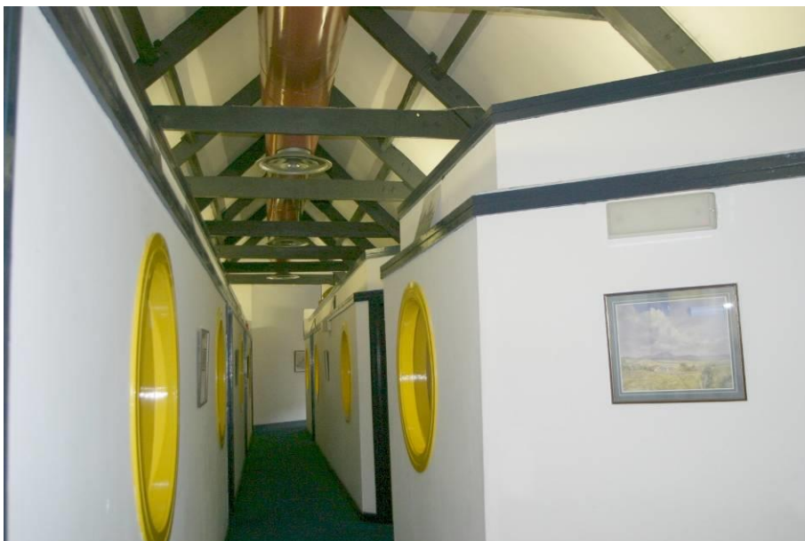
North section of the second floor, showing roof trusses.
