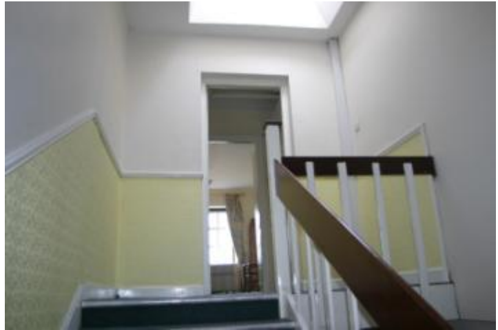
General views of the staircase.
