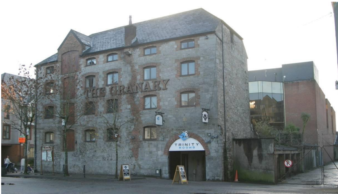
View of the granary building from Bank Place.
