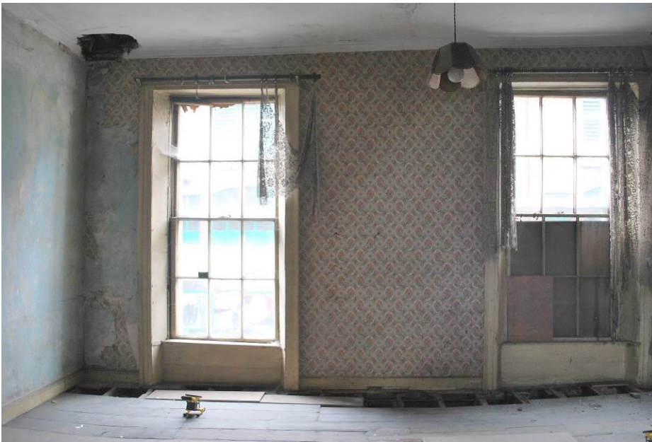
Fig. 5: Front room, first floor.
