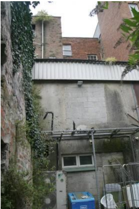
View of rear of No. 8 Rutland Street.
