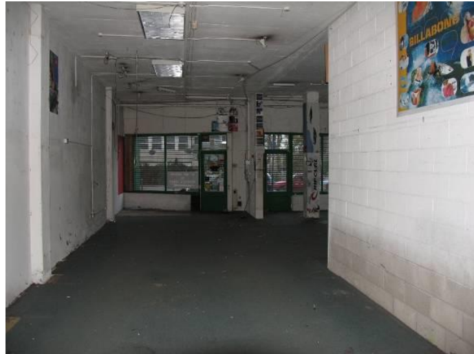
Views at ground floor level
