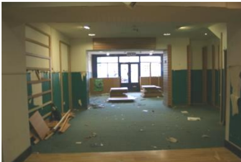
View of ground floor towards the front
