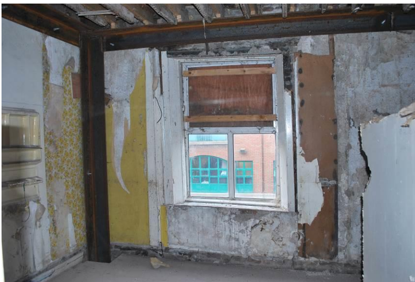
Fig. 5: Remedial works, second floor, front room.
