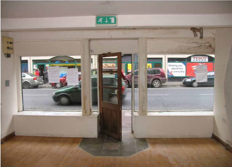
View of shop area, ground floor, towards the front of the building.
