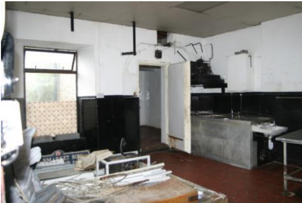
View of rear room and door through to area in return.
