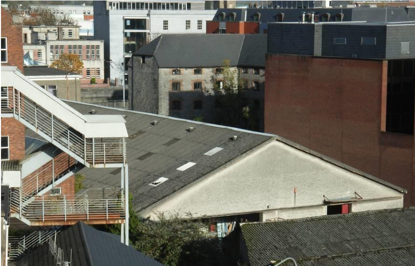
View from above showing the roof of the warehouse building.
