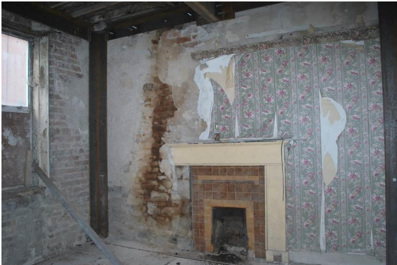
Fig. 4: Fireplace, first floor, front room.
