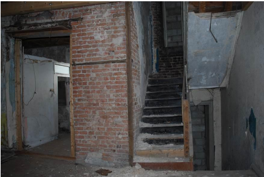
Fig. 7: Staircase, second floor.
