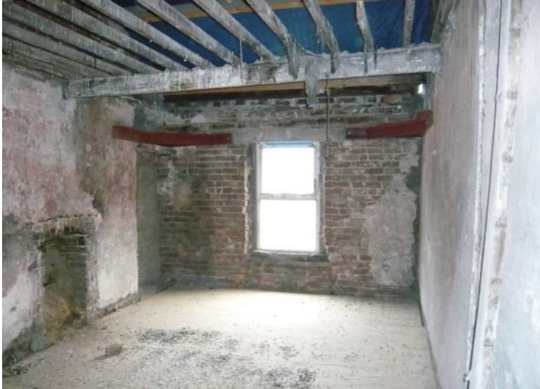
View to the front of the room.
