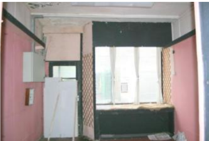
View towards front of front room, showing display window for shop.
