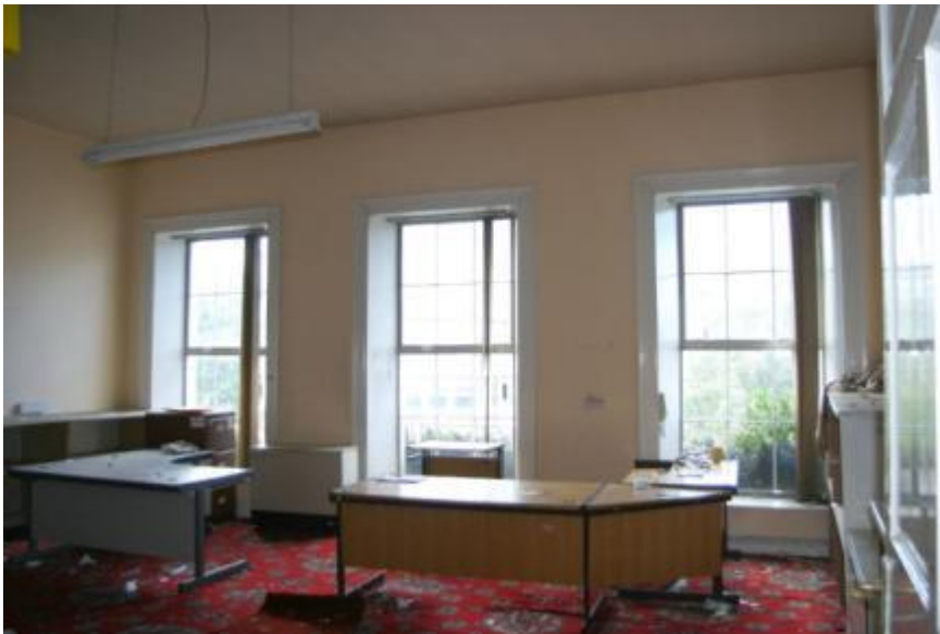
General view of front room.
