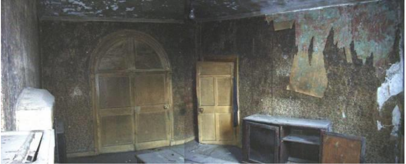
General view of rear room 1
