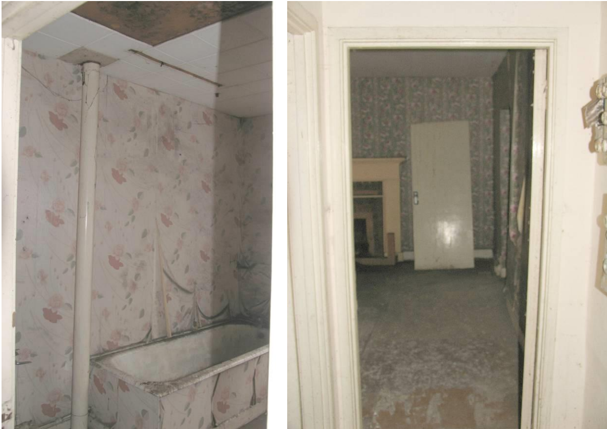
View of front rooms, bathroom and main living area, through modern partition and door.
