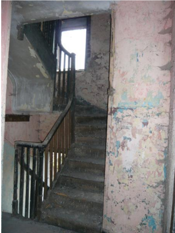
General view of staircase.
