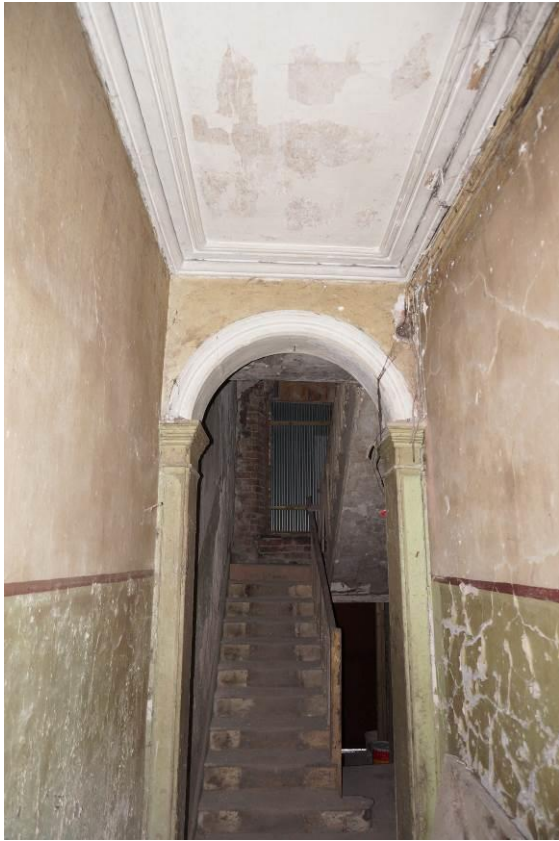
Fig. 6: Entrance hall and staircase.
