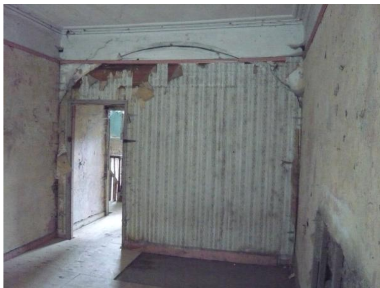
View to rear of room.
