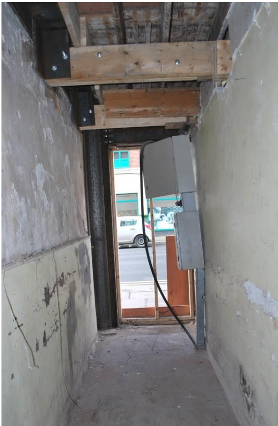
Fig. 1: Entrance hall, remedial works.
