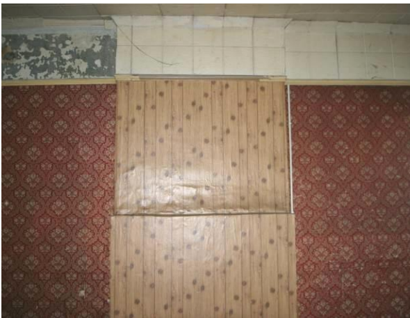
Chimney breast to front room.
