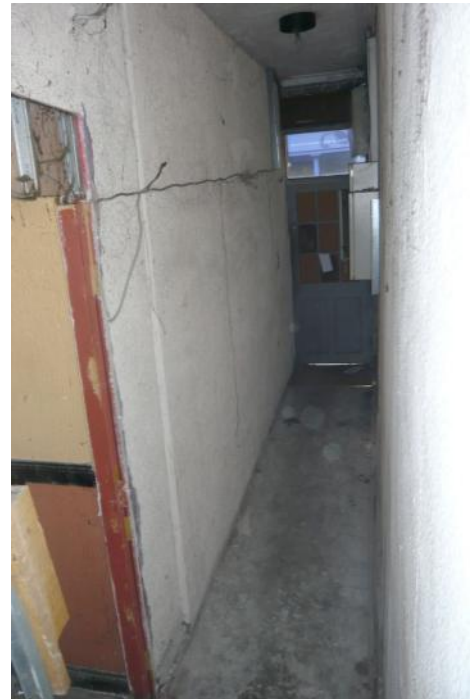
View of the hall and front door.
