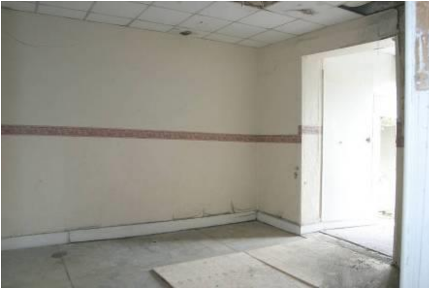
General view of rear room.
