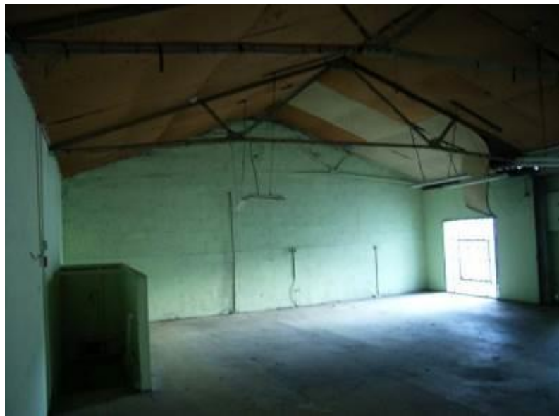
View showing steel truss
