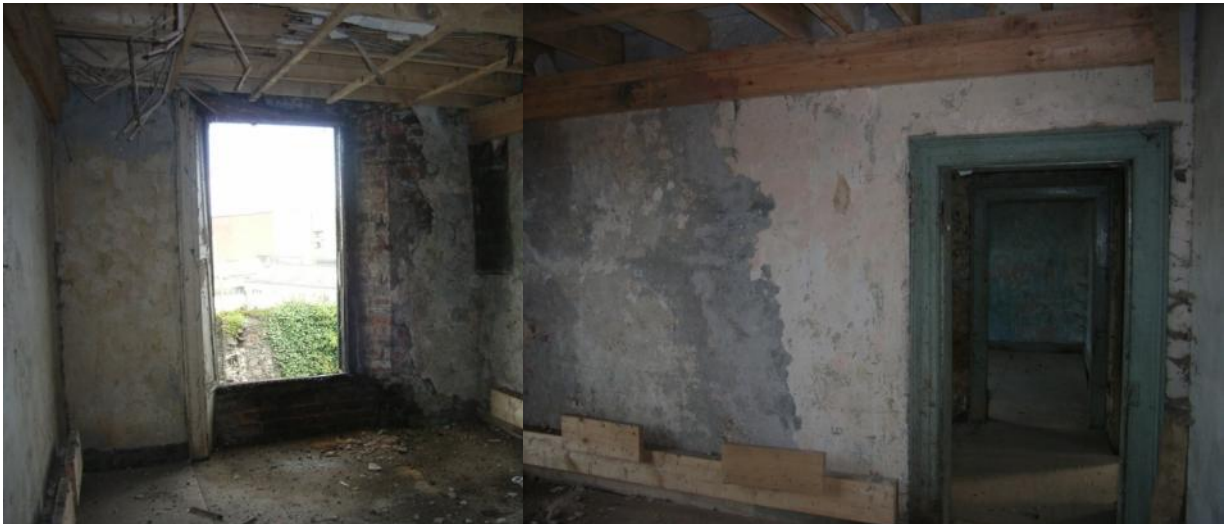
General view of the smaller rear room.
