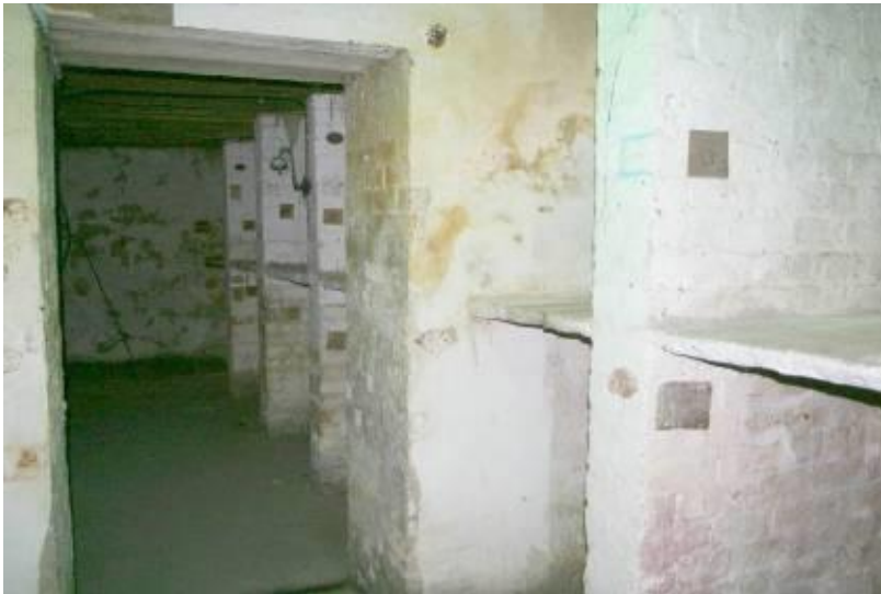
View of wine storage under Nos. 7 and 8 Ellen Street.
