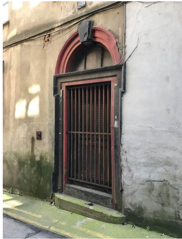
Fig. 7: Limestone doorcase to laneway.
