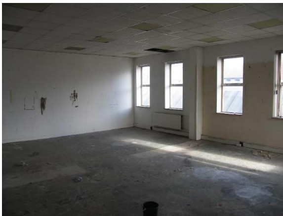
First floor facing rear façade
