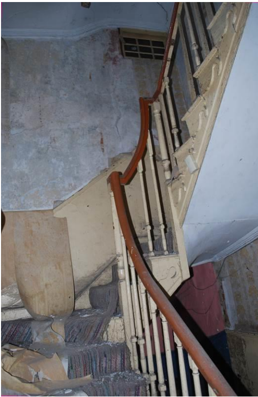
Fig. 6: centrally located staircase
