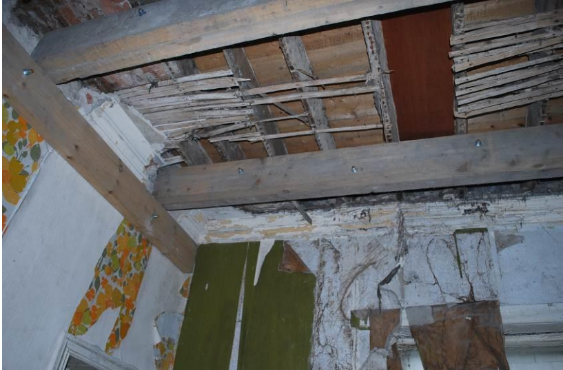
Fig. 3: Remedial works, propping of floors, first floor.
