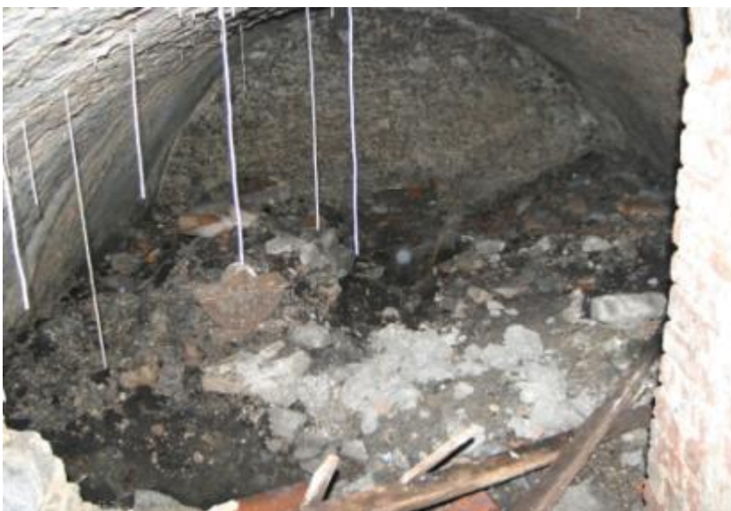
View of the accessible cellar below Rutland Street.
