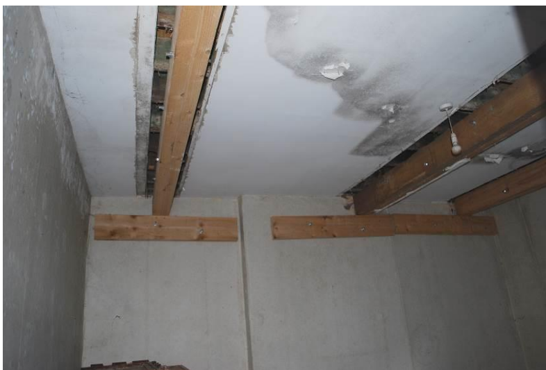
Fig. 2: Remedial structural works, rear room, 2 nd floor.
