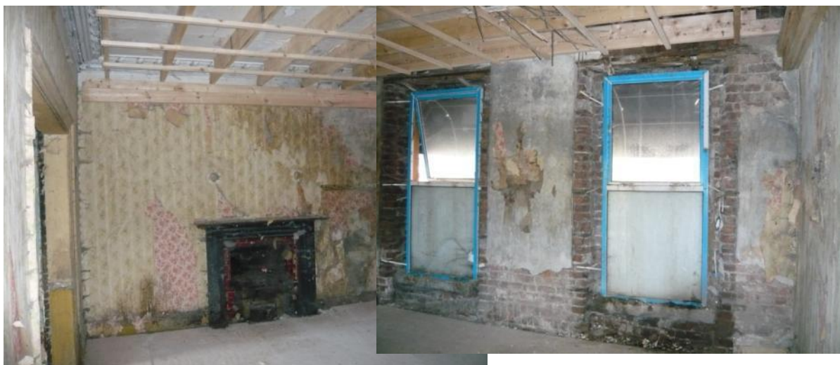
View of the front room, showing the fireplace and windows.
