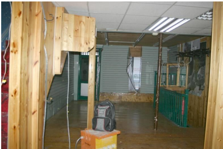
View towards shopfront.
