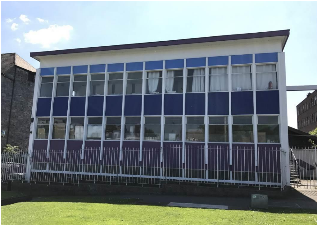
Fig. 1: Bank Place elevation.
