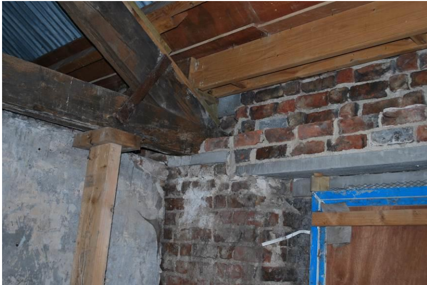
Fig. 1: Parapet rebuilt, new window head. Second floor, front façade.
