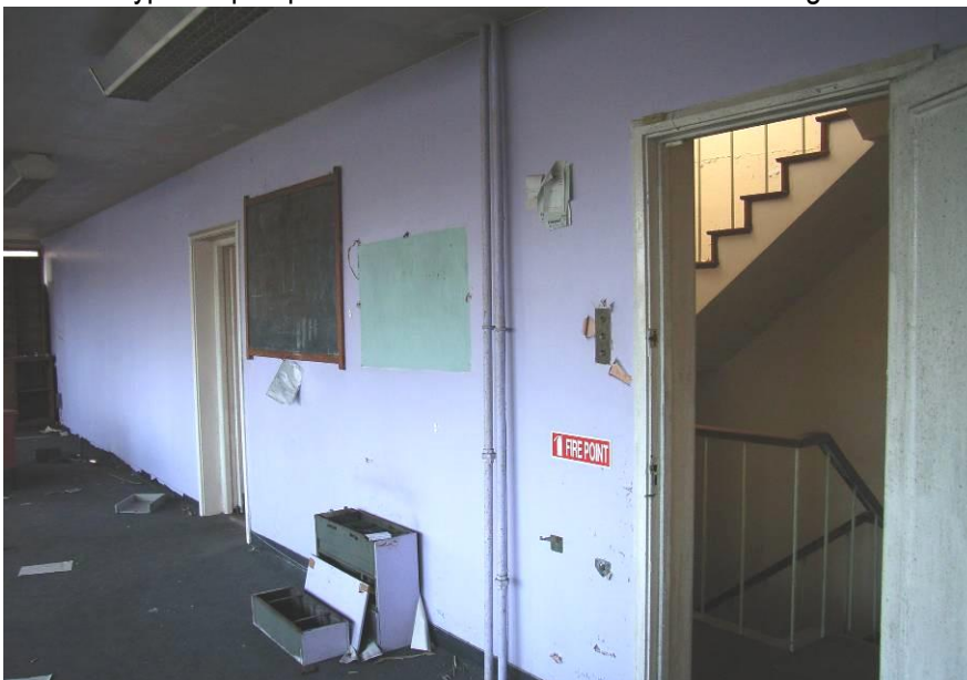
Internal wall to office area, showing access to stairwell.
