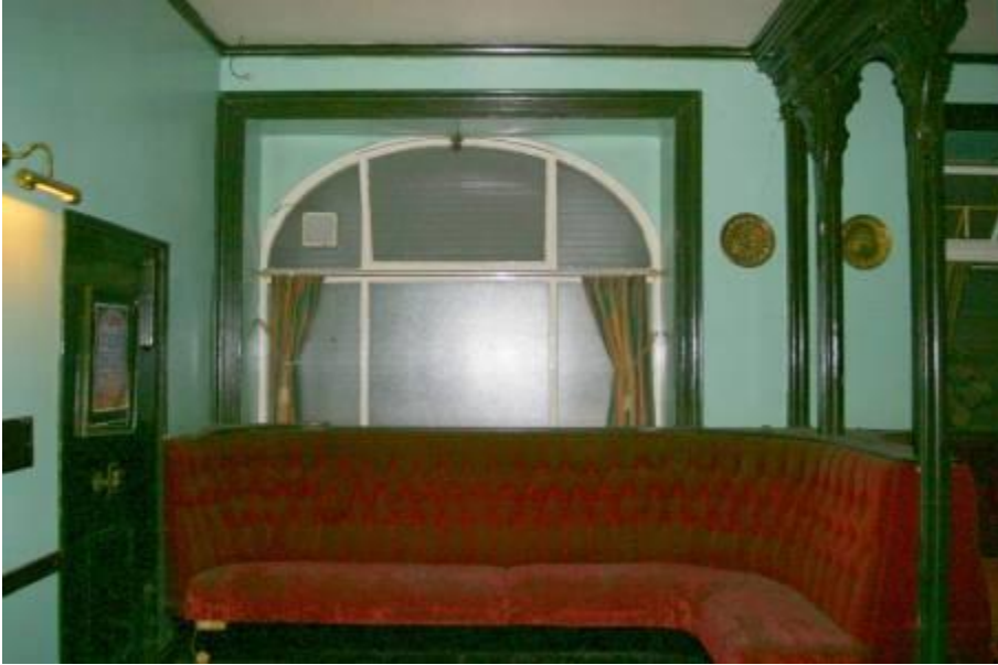
Large timber window located in former carriage arch to central bay of building.
