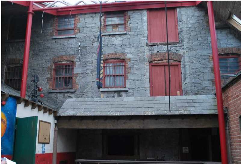
Fig. 4: Timber sash windows.
